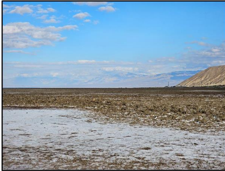
Figure 3: The drill rig on the first drill hole as seen from the second hole site at the Liberty Lithium Brine Project
