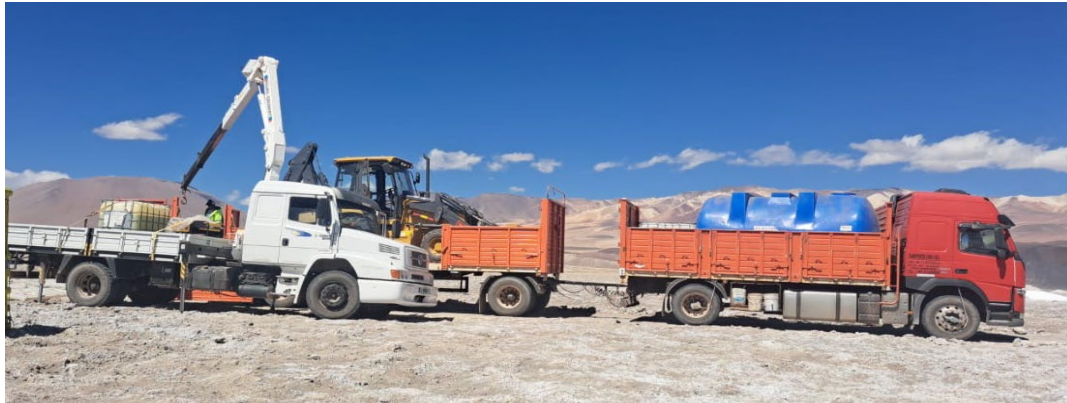
Figure 2 – Equipment trucks carrying front end loaders and initial drilling supplies arrive at Rio Grande Sur.
