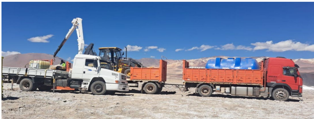
Figure 2 – Equipment trucks carrying front end loaders and initial drilling supplies arrive at Rio Grande Sur.
