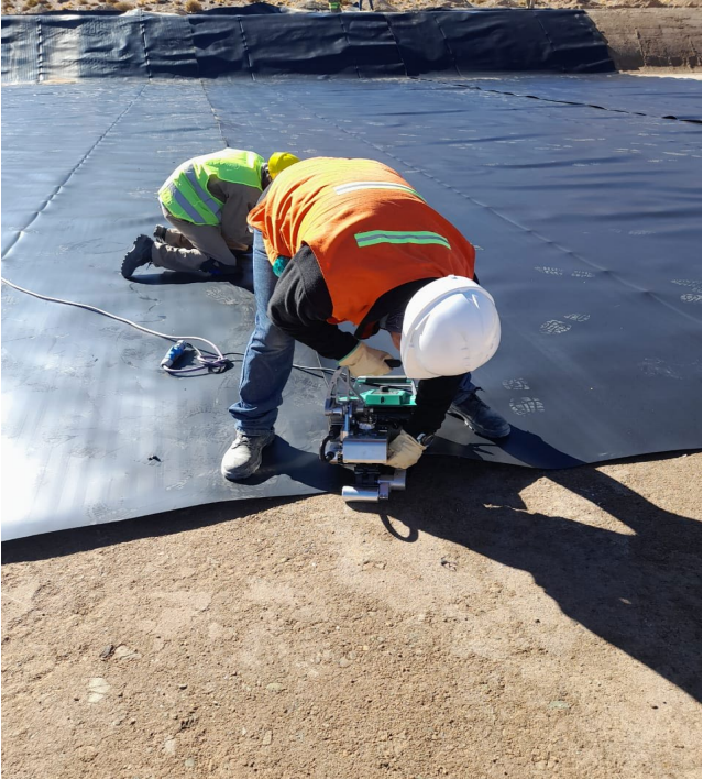
Figures 4 and 5 - Liner installation process Pond 1
