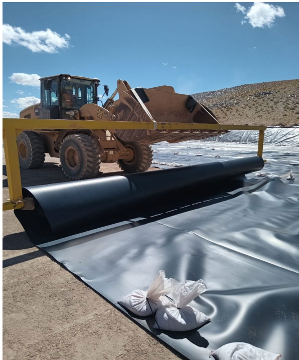
Figures 4 and 5 - Liner installation process Pond 1
