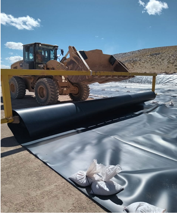
Figures 4 and 5 - Liner installation process Pond 1
