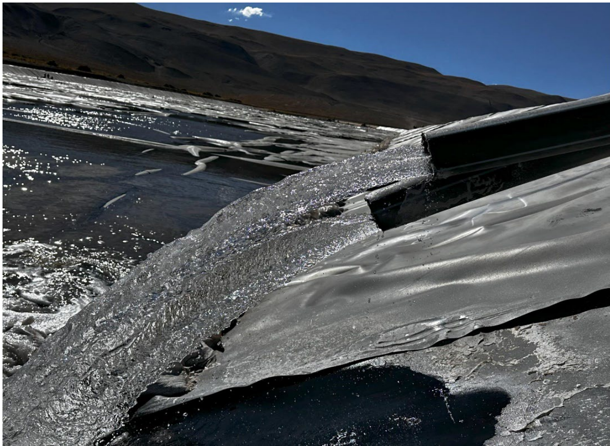
Figure 3 – The commencement of the filling of Pond 1
