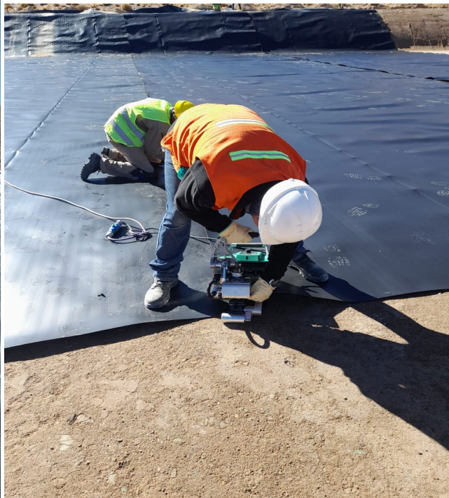
Figures 4 and 5 - Liner installation process Pond 1
