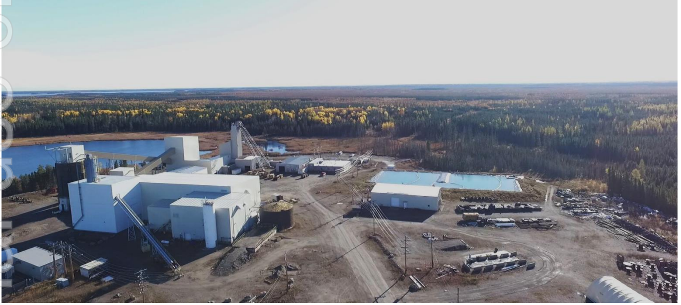
Figure 1: Wabowden Project - Bucko Mine and Processing Facility
