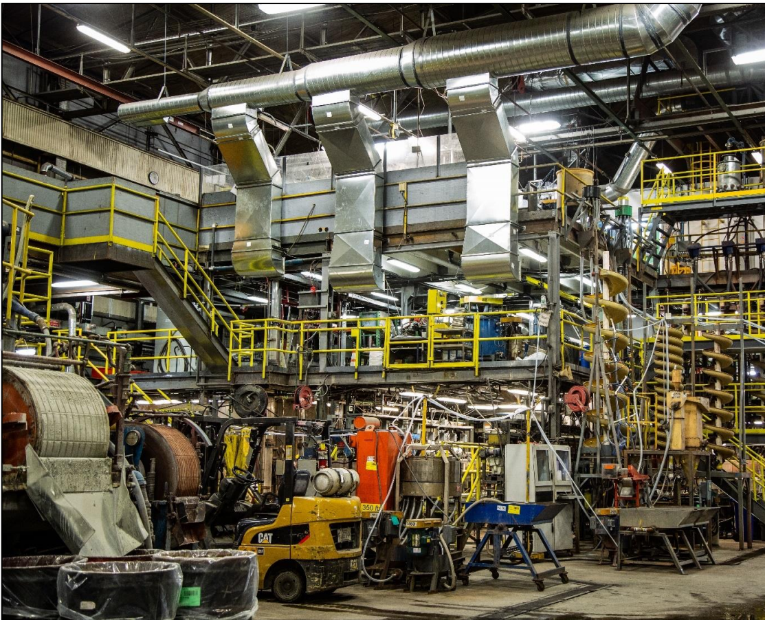
Iron Bear pilot plant setup at COREM facilities
