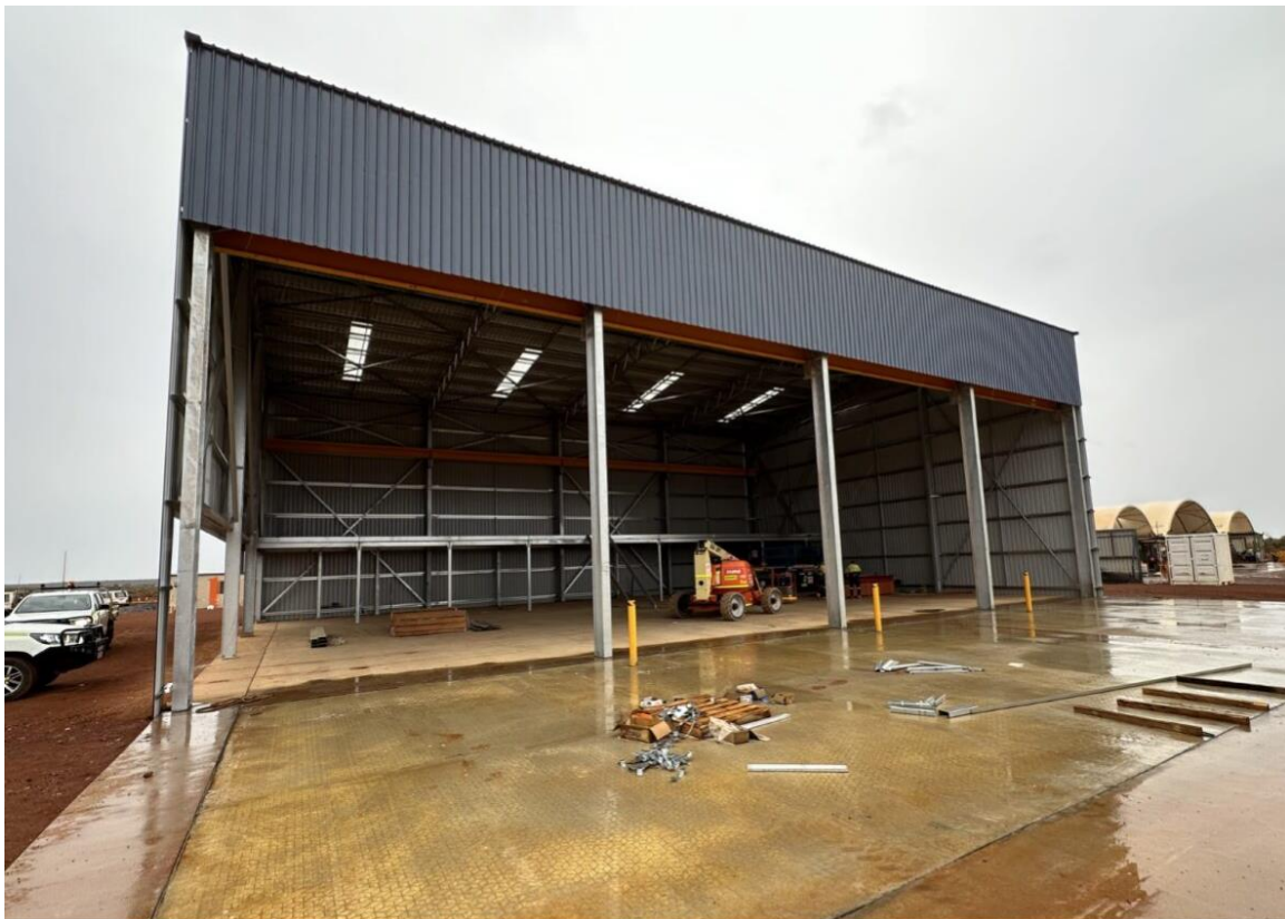
Figure 10 – Underground Heavy Vehicle workshop under construction.
