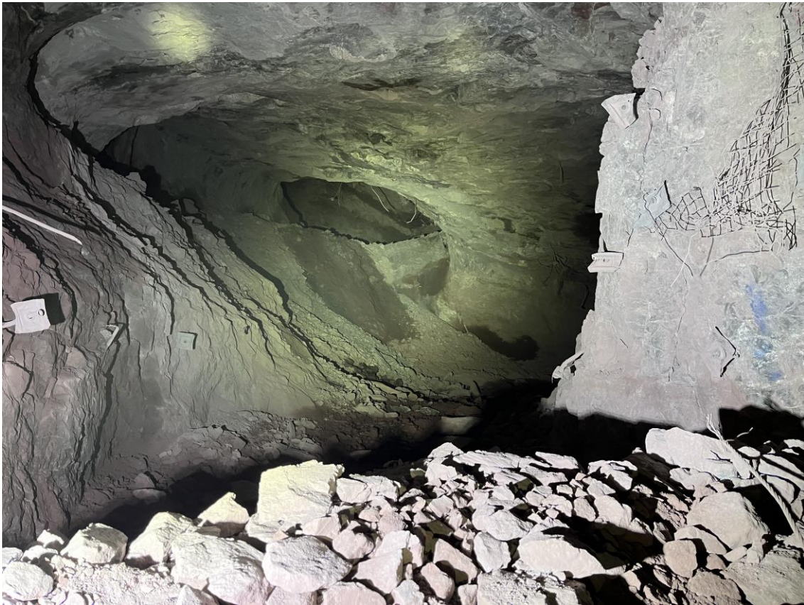
Figure 9 – Underground Apron stope at Abra (December 2023).
