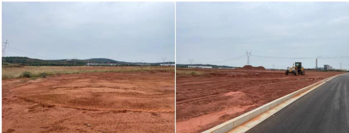
Image 2 and 3: Firebird's industrial land for its Sulphate Plant at Jinshi Chemical Park
