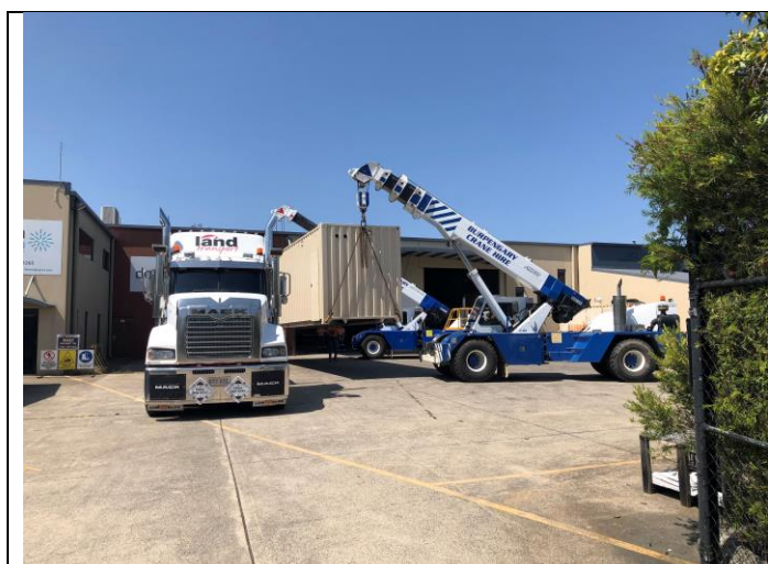
Image 1) De.mem Containerized Membrane Based Water Treatment Plant Being Shipped to Mining Site
