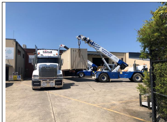
Image 1) De.mem Containerized Membrane Based Water Treatment Plant Being Shipped to Mining Site
