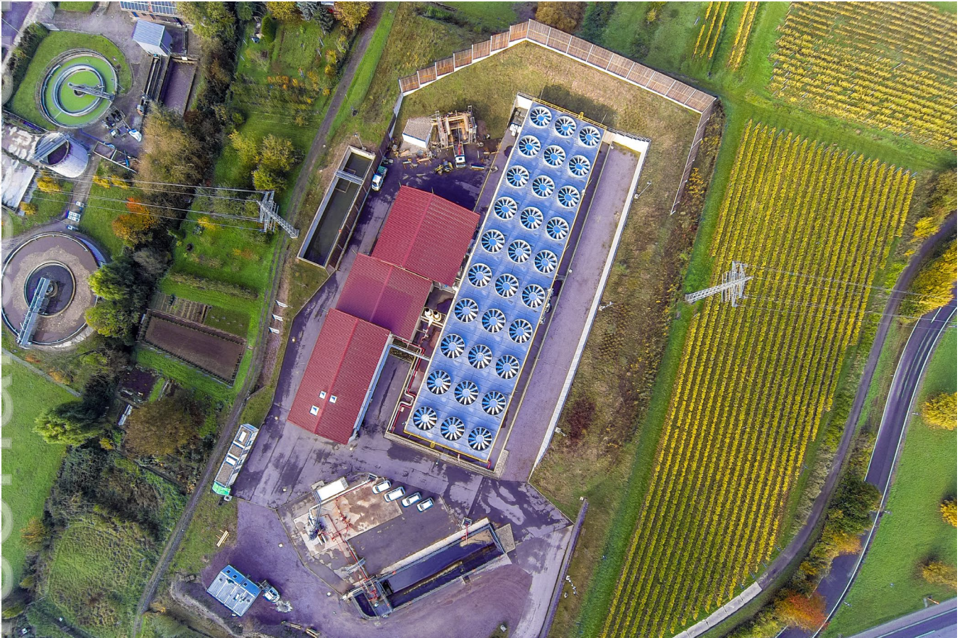
Figure 1 Vulcan's Natürlich Insheim geothermal renewable energy wells and plant
