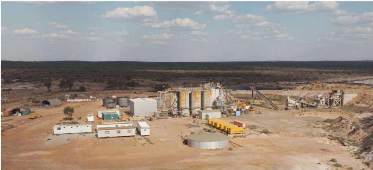
Figure 7 - Brightstar Plant looking from the northwest.
