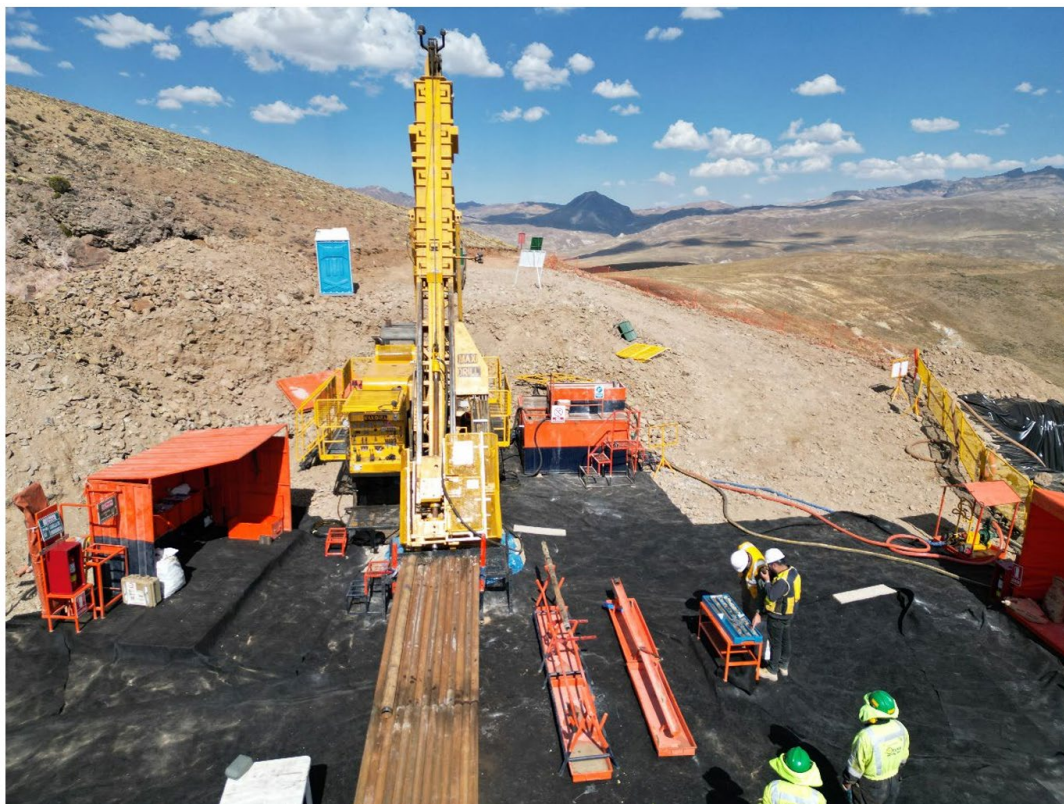
Figure 1: Drill rig on site at Cobremani target
