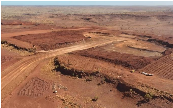
Ken's Bore pit
