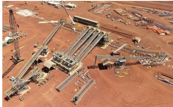
Ken's Bore crushing plant works
