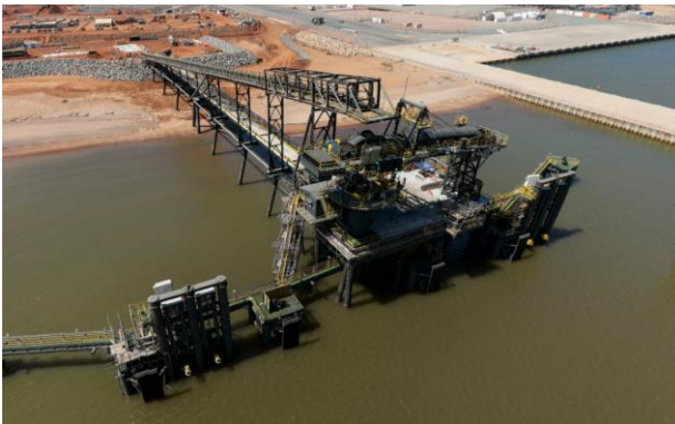
Transhipping wharf at Port of Ashburton
