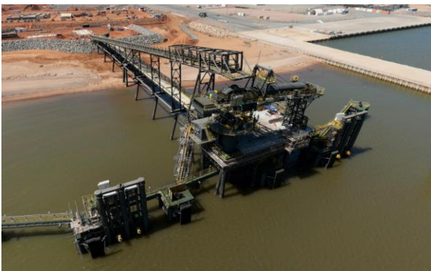
Transhipping wharf at Port of Ashburton
