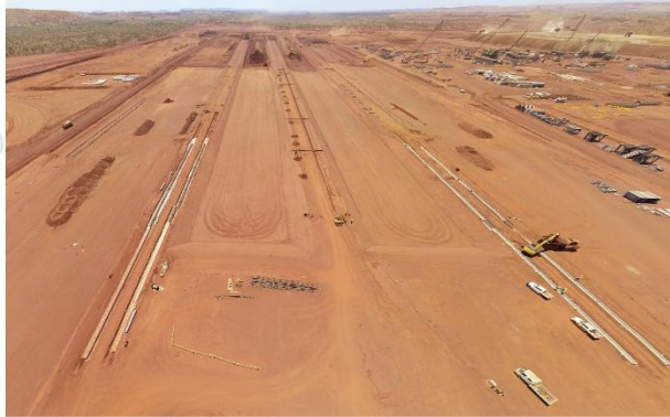
Stacker works and stockyard earthworks
