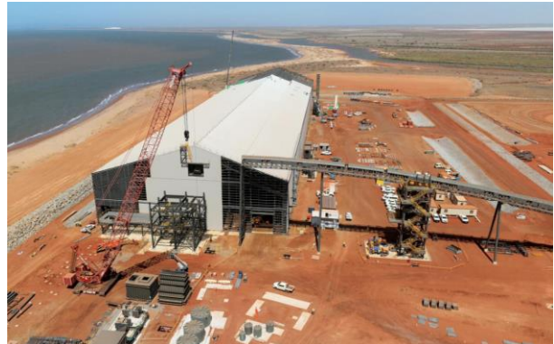
Port of Ashburton ore storage shed
