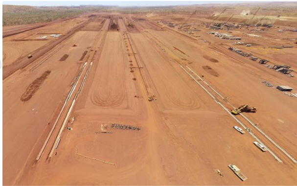
Stacker works and stockyard earthworks
