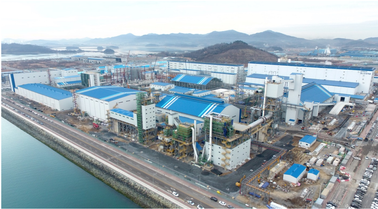
Figure 1: The PPLS LHM facility as at 17 January 2024.
