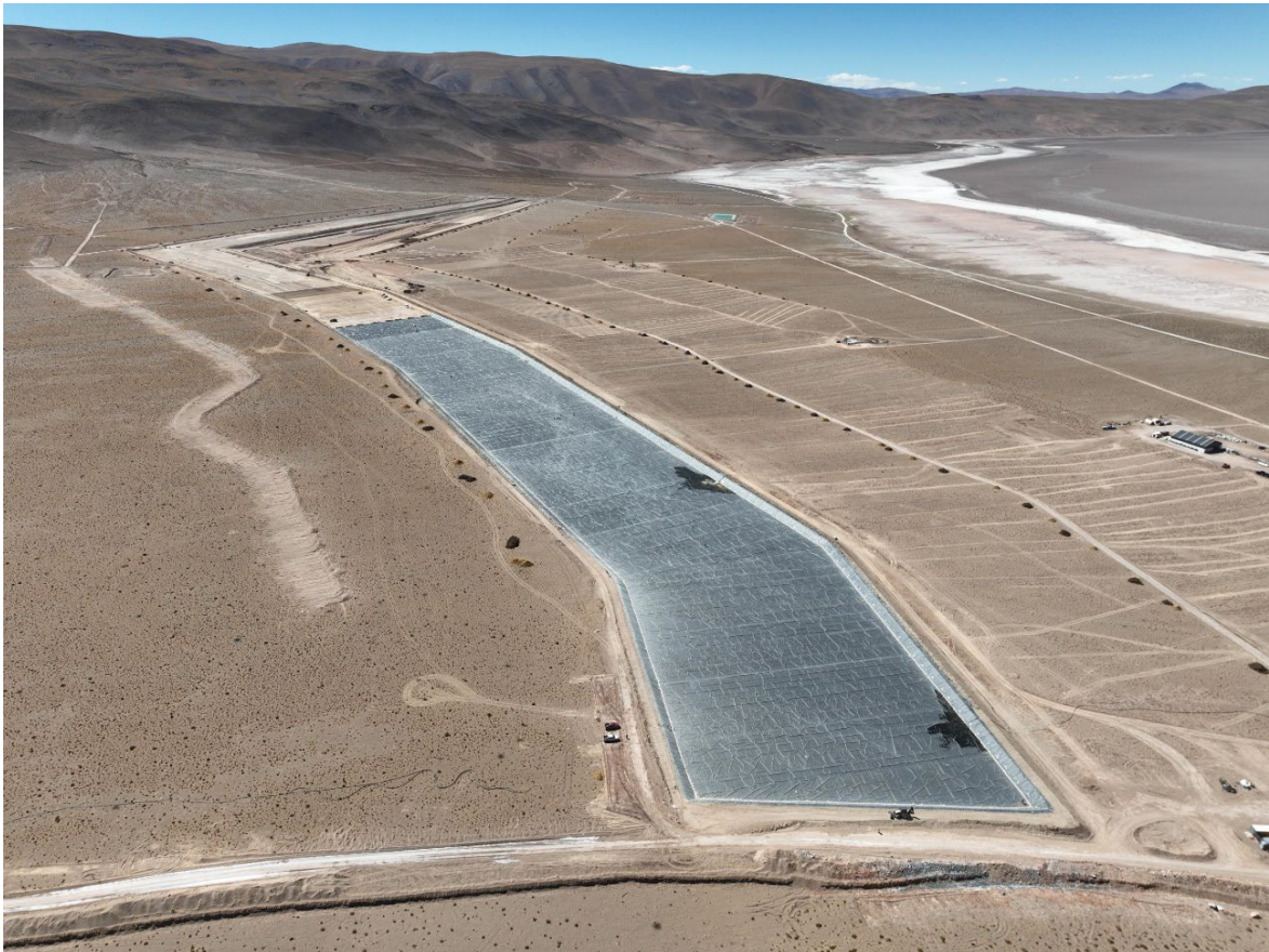
The overall progression of liner installation on Pond 1
