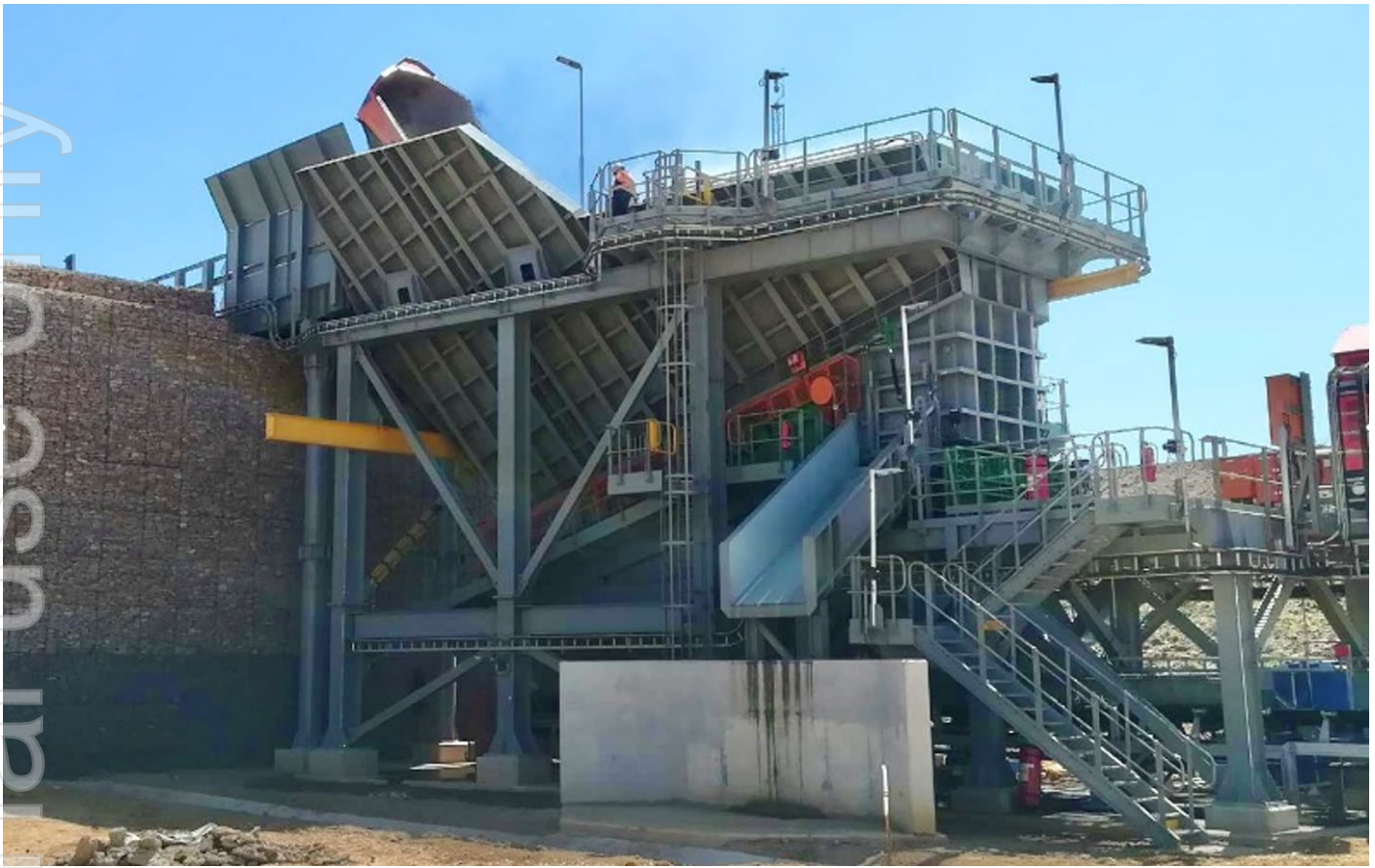
Figure 9. Feed Hopper and Mineral Sizer
