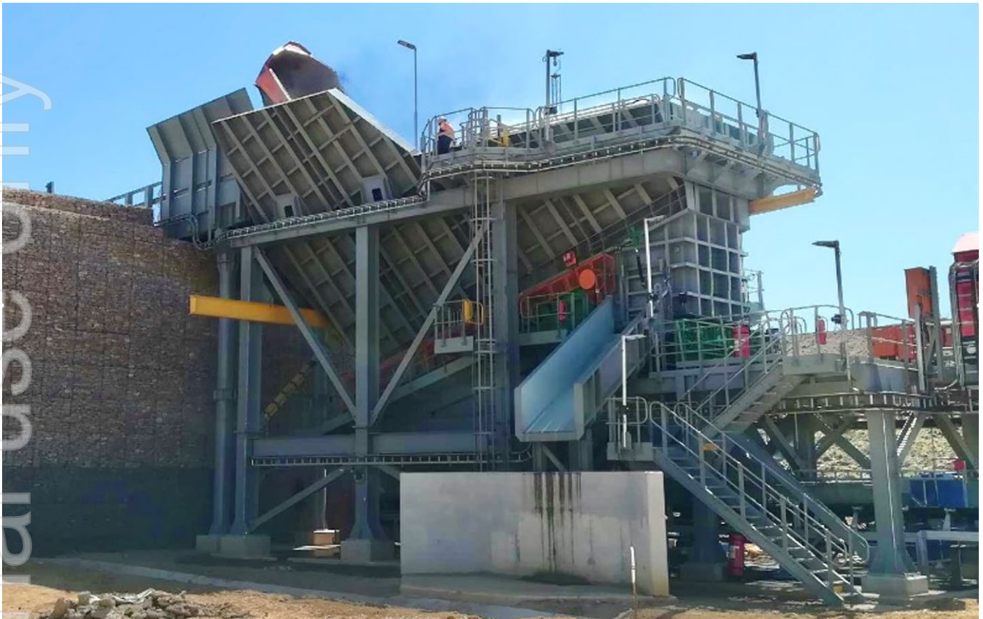
Figure 9. Feed Hopper and Mineral Sizer
