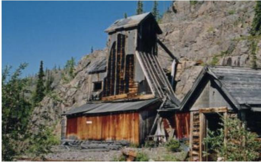
Photo 2 Contact Lake Mine headframe, July 2005.
