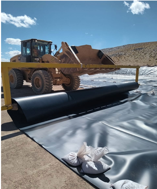
Liner installation process
