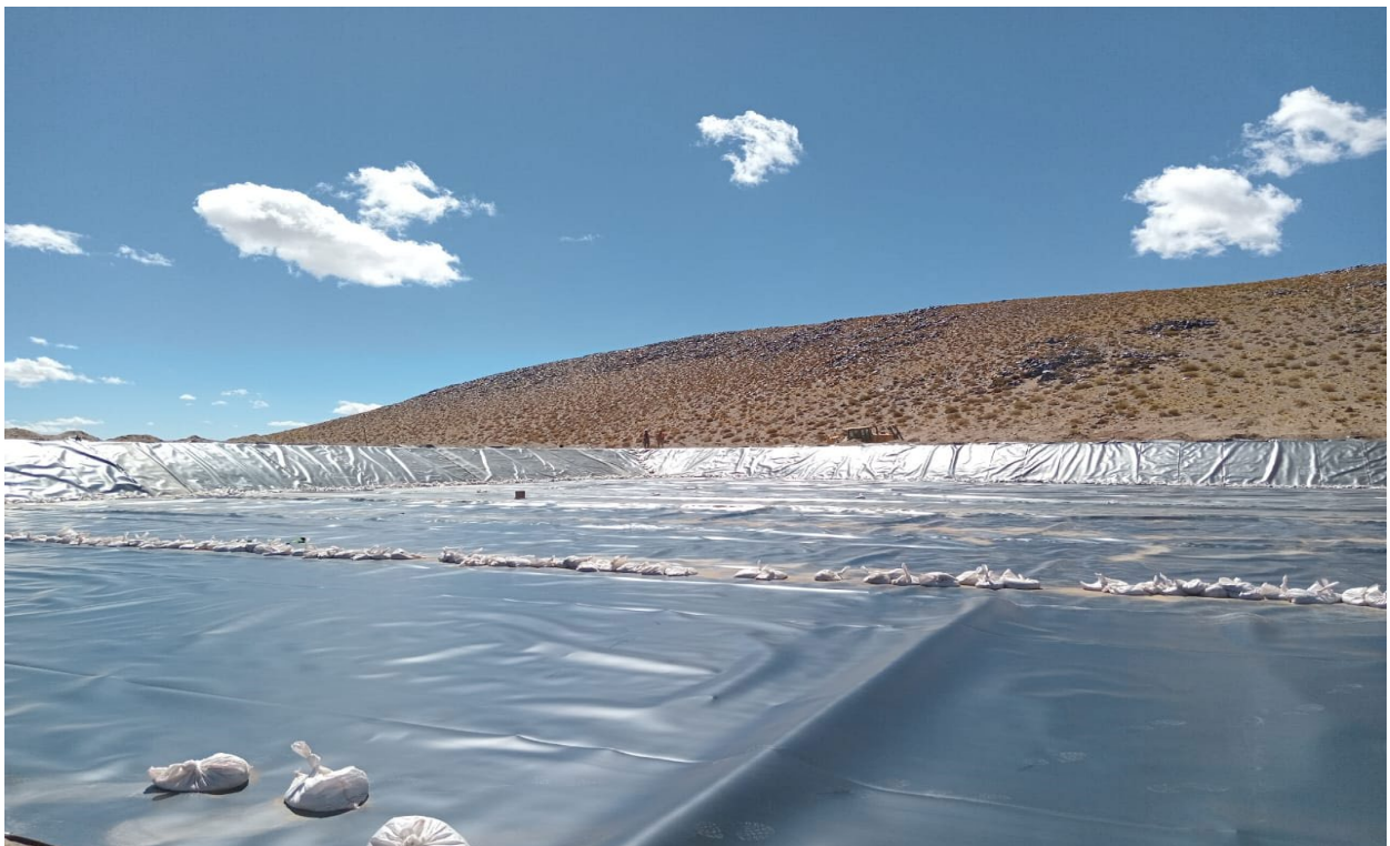
Liner installation commencement
