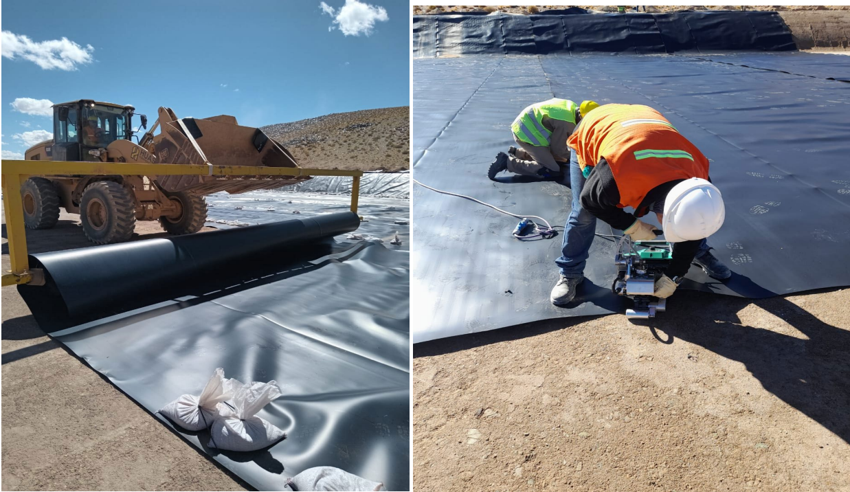
Liner installation process
