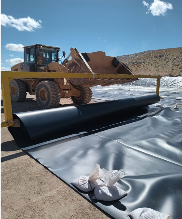
Liner installation process
