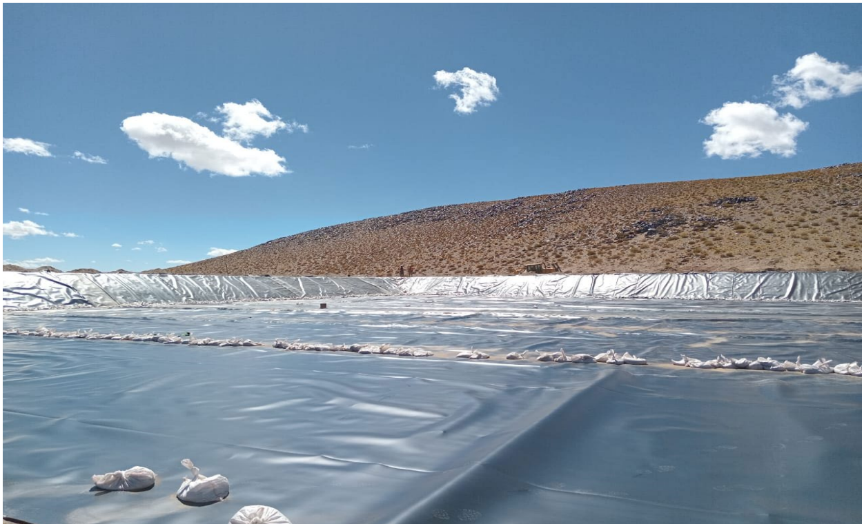
Liner installation commencement
