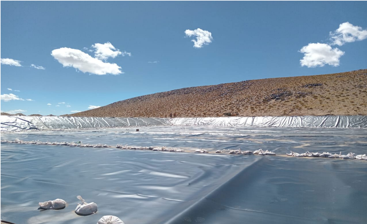
Liner installation commencement
