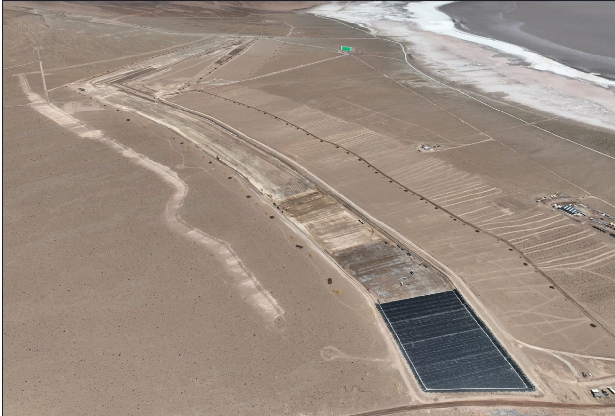
Overall progression of liner installation on Pond 1
