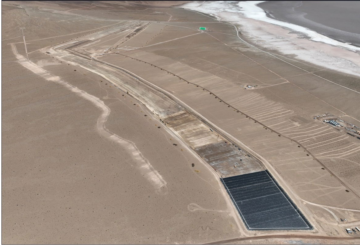
Overall progression of liner installation on Pond 1
