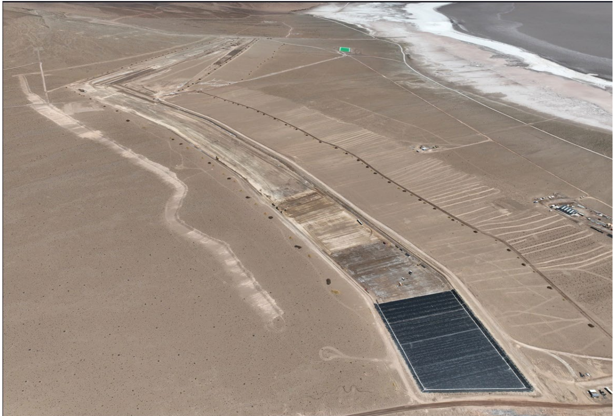
Overall progression of liner installation on Pond 1
