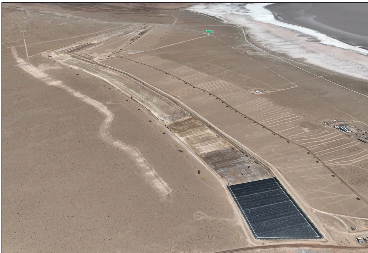
Overall progression of liner installation on Pond 1
