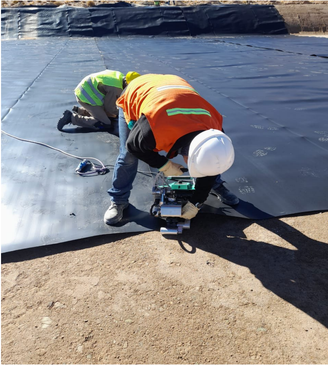
Liner installation process
