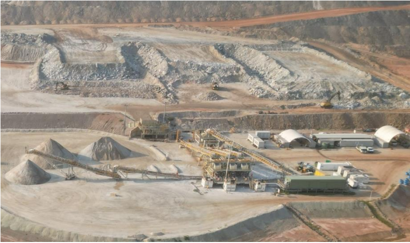
Crushed stockpiles (foreground) and ROM stockpiles (background) December 2023
