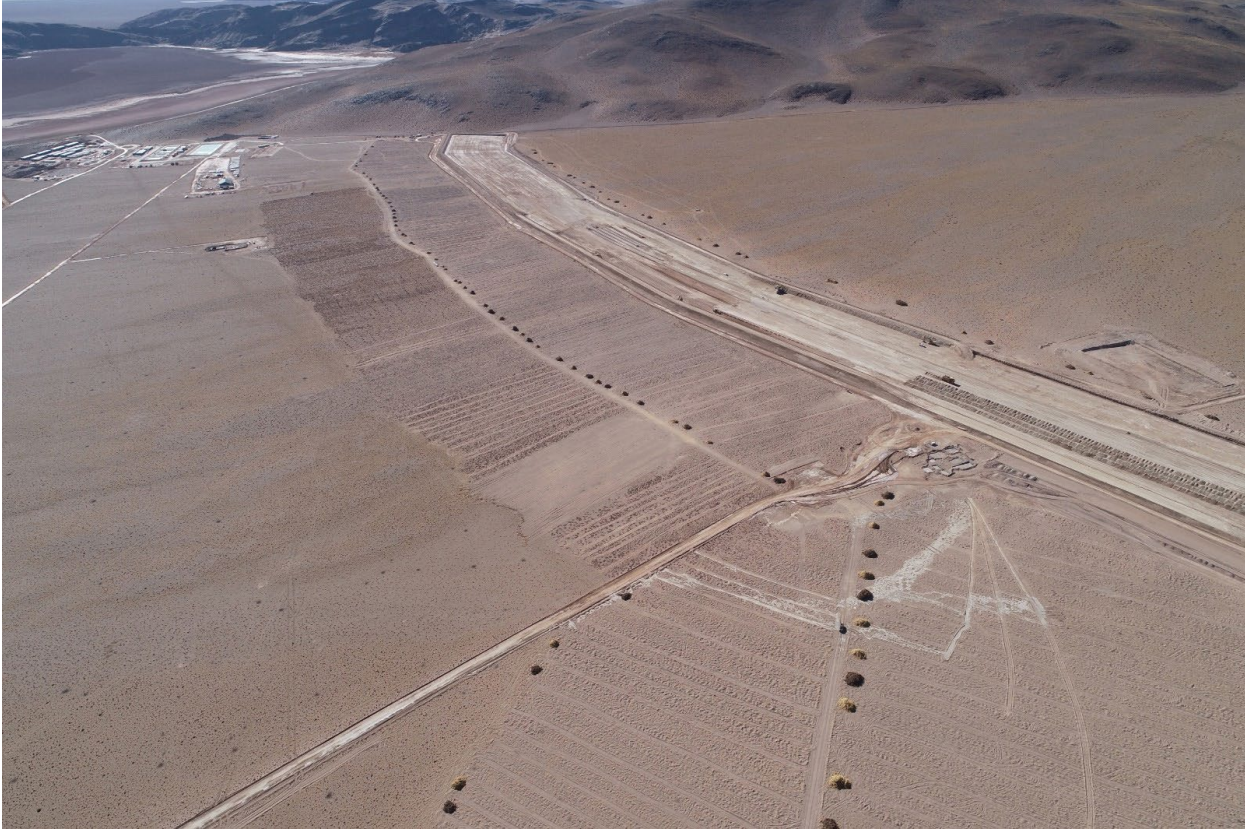
Overhead view of HMW development
