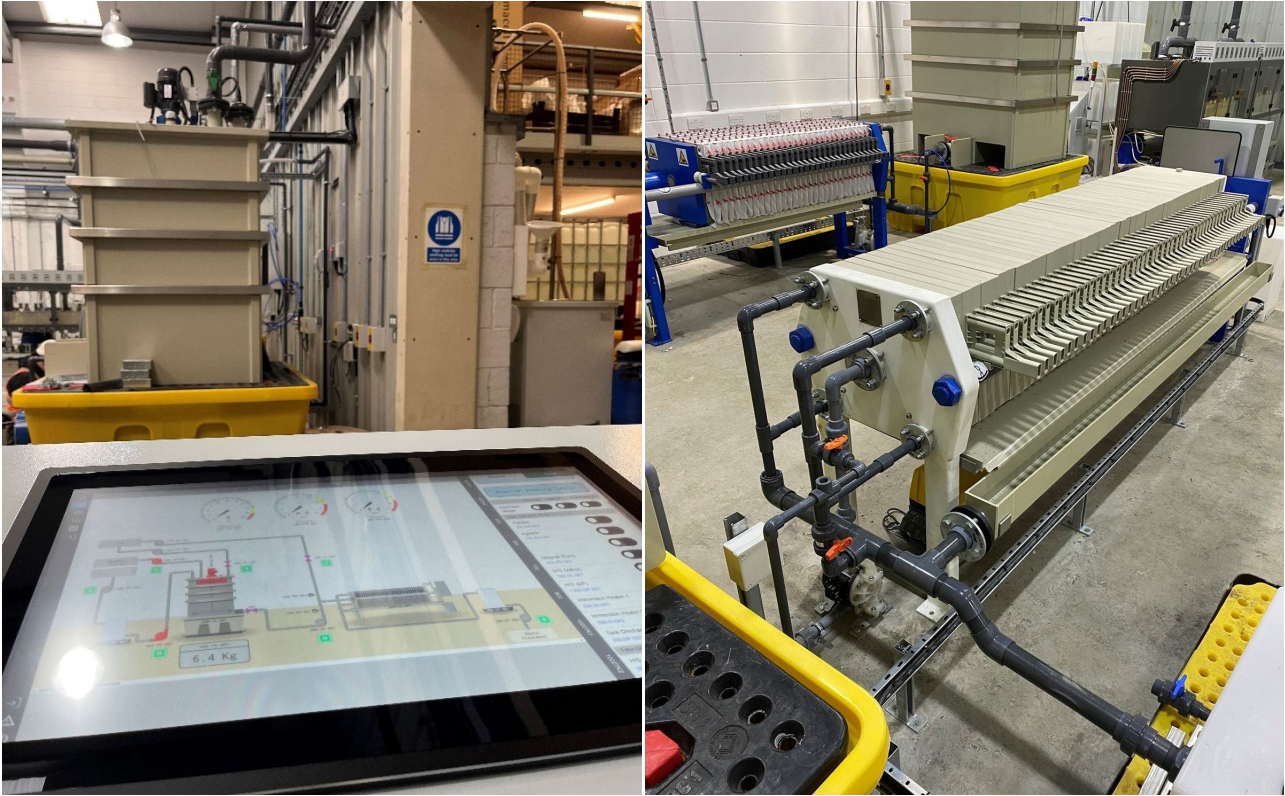
Figure 3: Left, Scada control panel in front of reactor vessel, and right, new digestion product filter.
