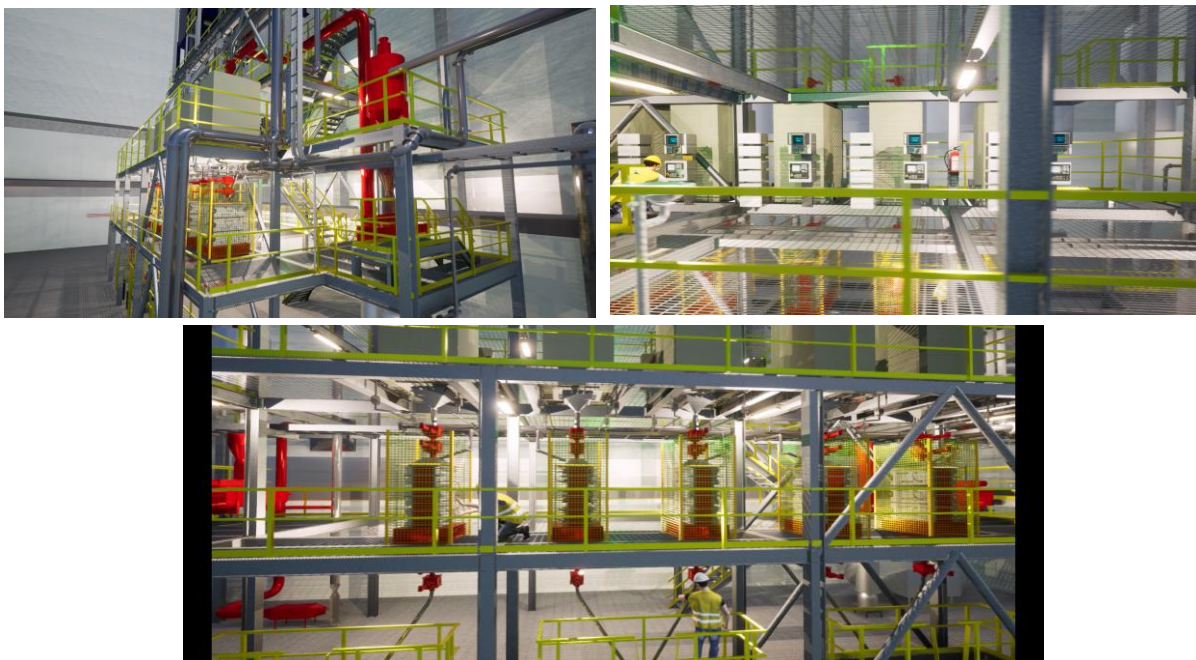
Figure 6 – In-house designed packed bed calciners
