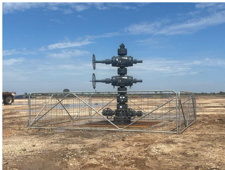
Wellhead installed at Daydream-2
