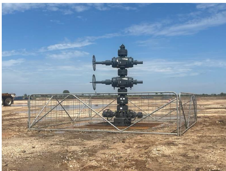
Wellhead installed at Daydream-2
