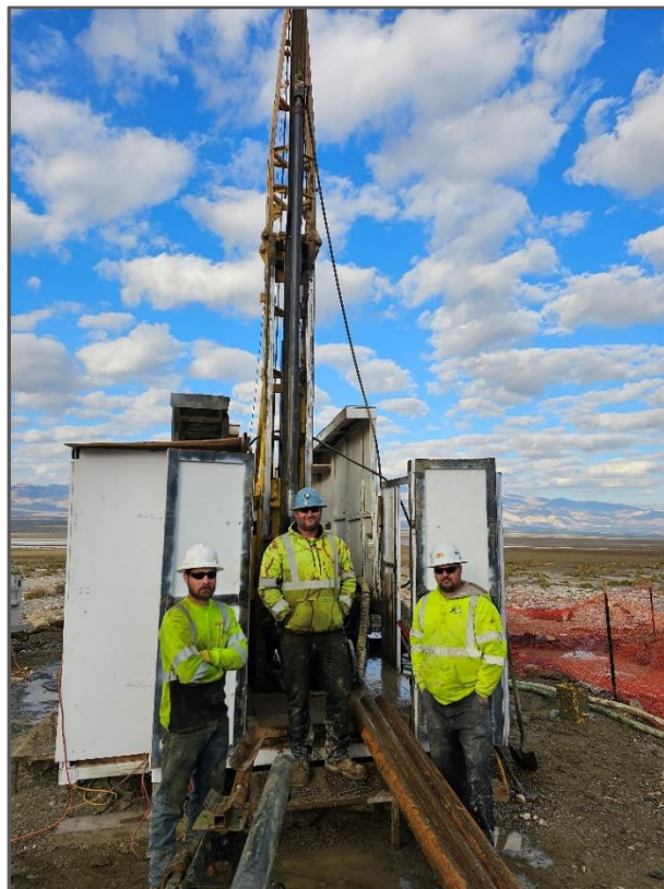
Figure 3: Drill rig at the first drill hole at the Liberty Lithium Brine Project
