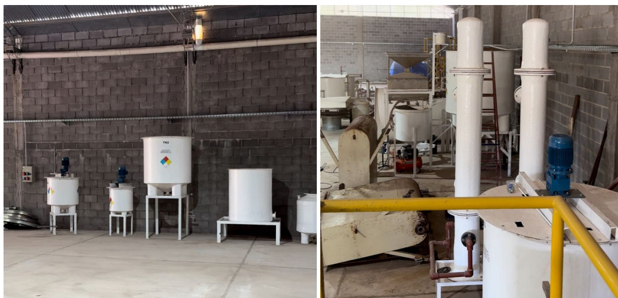
Figure 1 – Plant mixing tanks and columns being refurbished at the new Pursuit Lithium Facility in Salta, Argentina.
