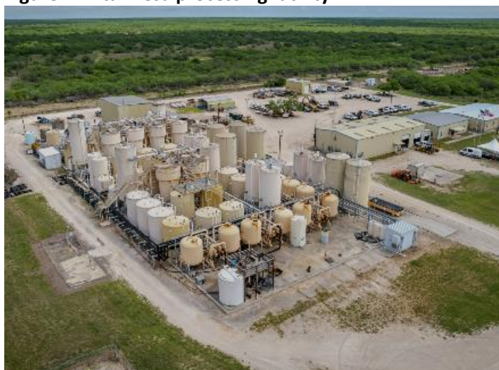
Figure 2: Alta Mesa processing facility
