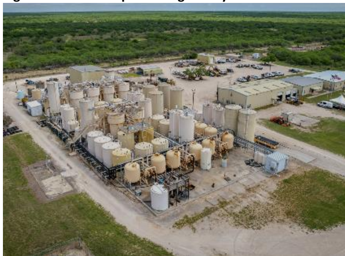
Figure 2: Alta Mesa processing facility
