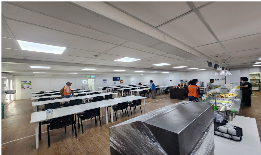
Figure 5: New camp mess nearing completion
