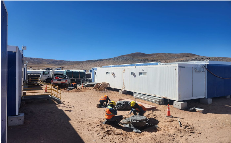
Figure 4: Camp infrastructure and services being installed
