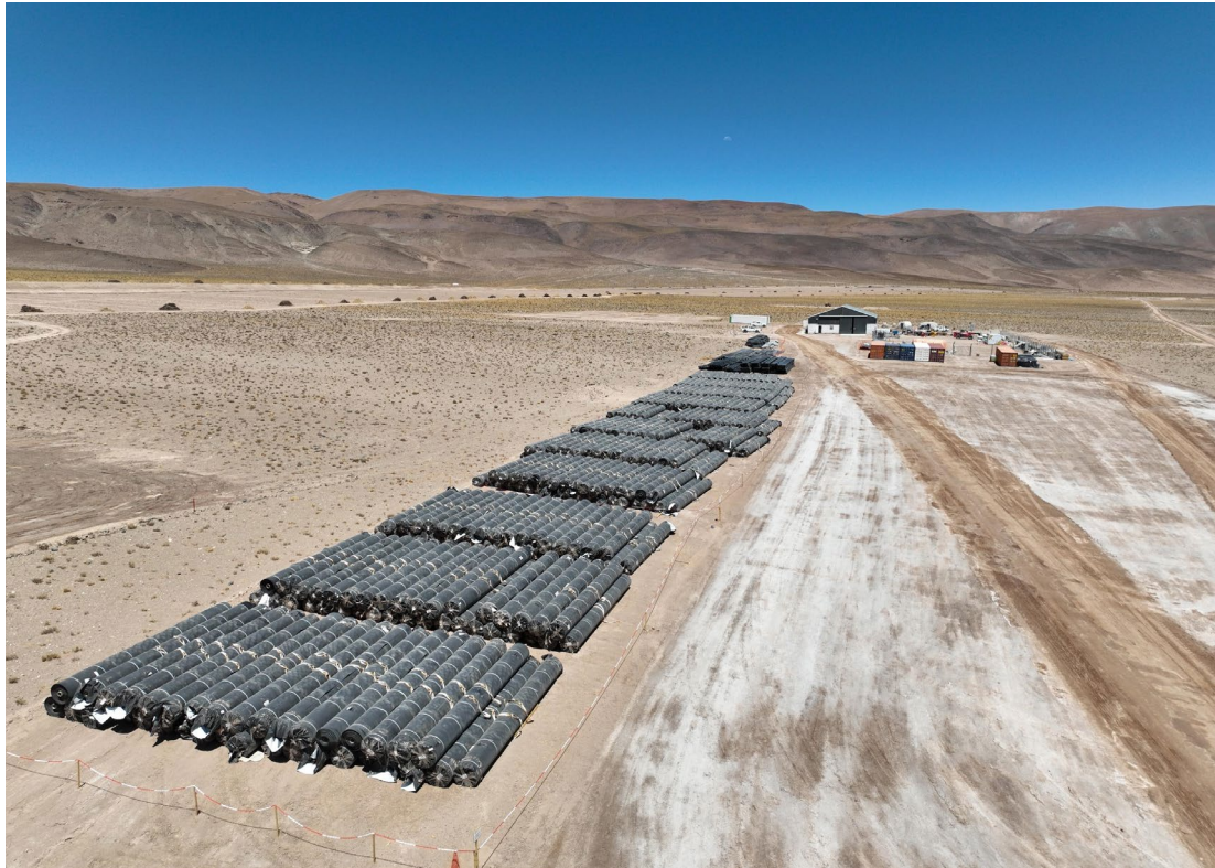
Figure 6: Liners on site ready for installation
