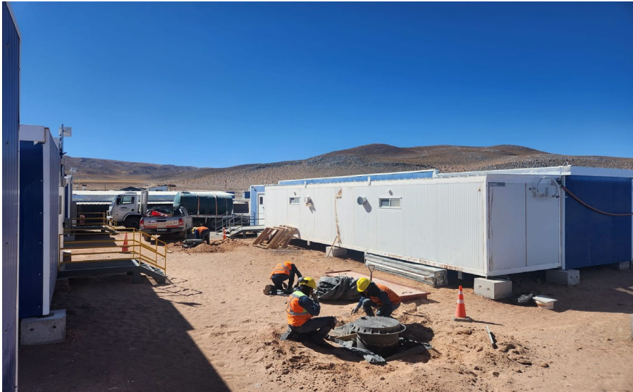
Figure 4: Camp infrastructure and services being installed
