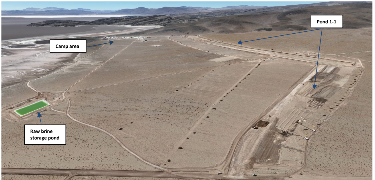
Figure 1: Pond 1 construction progress and Ponds 2 & 3 preparation works underway
