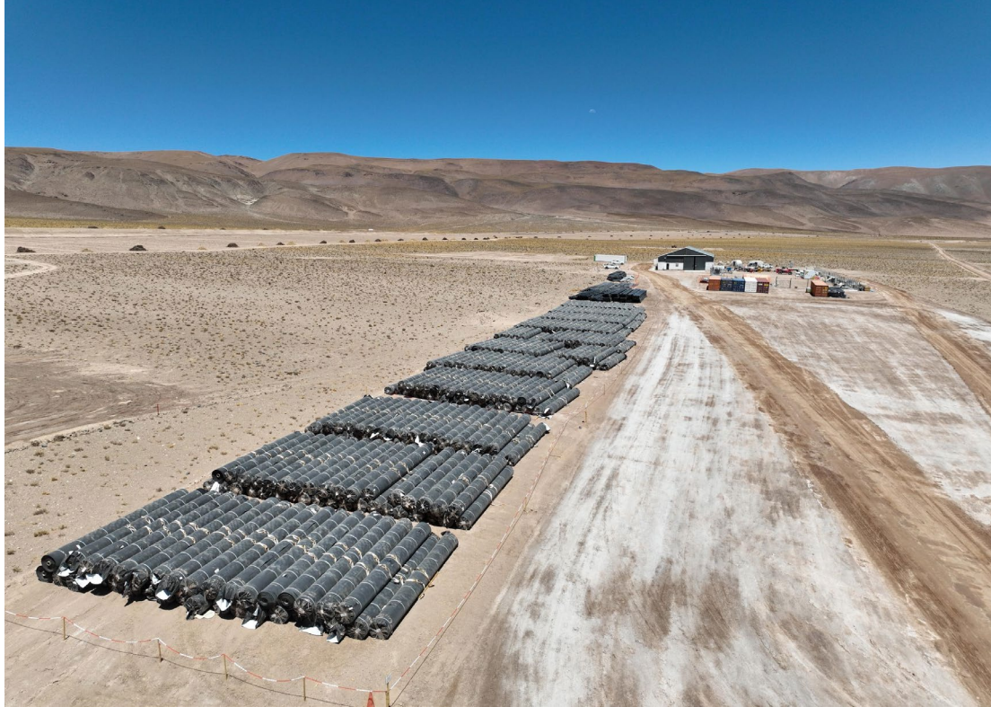
Figure 6: Liners on site ready for installation
