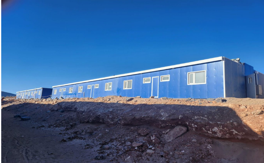
Figure 3: Camp modules installed
