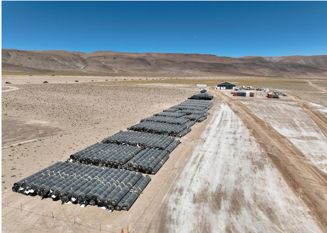
Figure 6: Liners on site ready for installation
