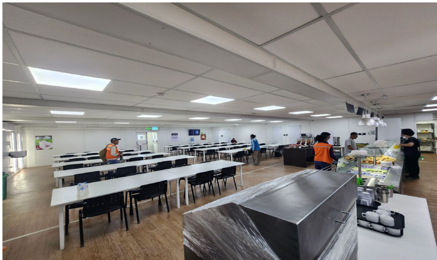
Figure 5: New camp mess nearing completion
