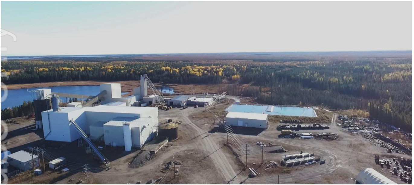
Figure 1: Wabowden Project - Bucko Mine and Processing Facility
