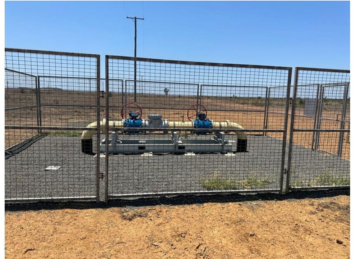
Installed tie in point to collect waste mine gas
