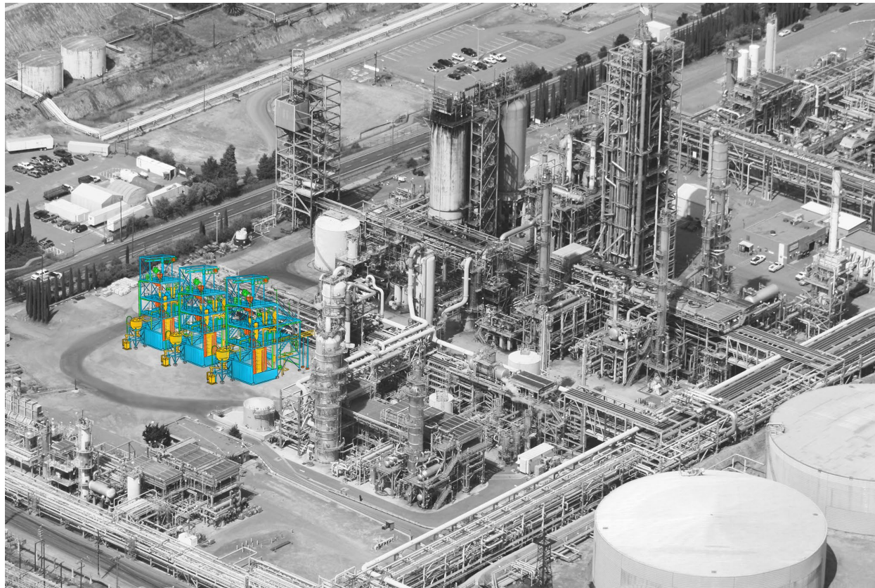
Conceptual design of Hazer facility co-located with 3 rd party refinery (Source: stock image not Hazer infrastructure)
