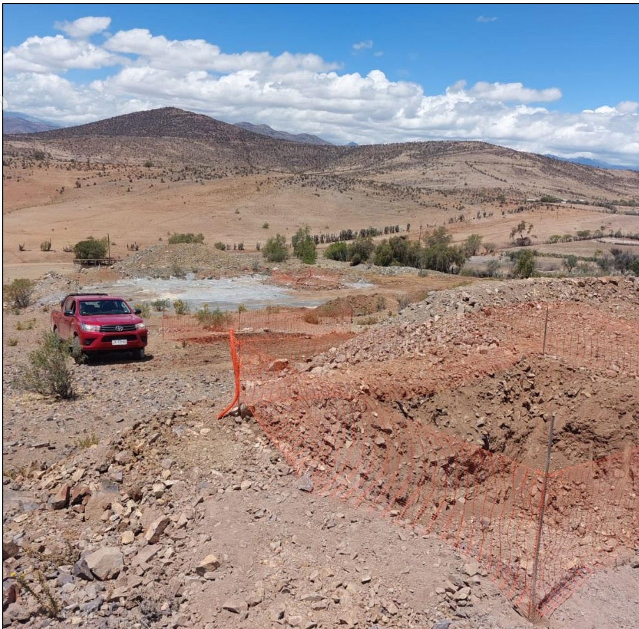
Figure 4: Drill pads constructed at the high priority El Quillay drill target.
