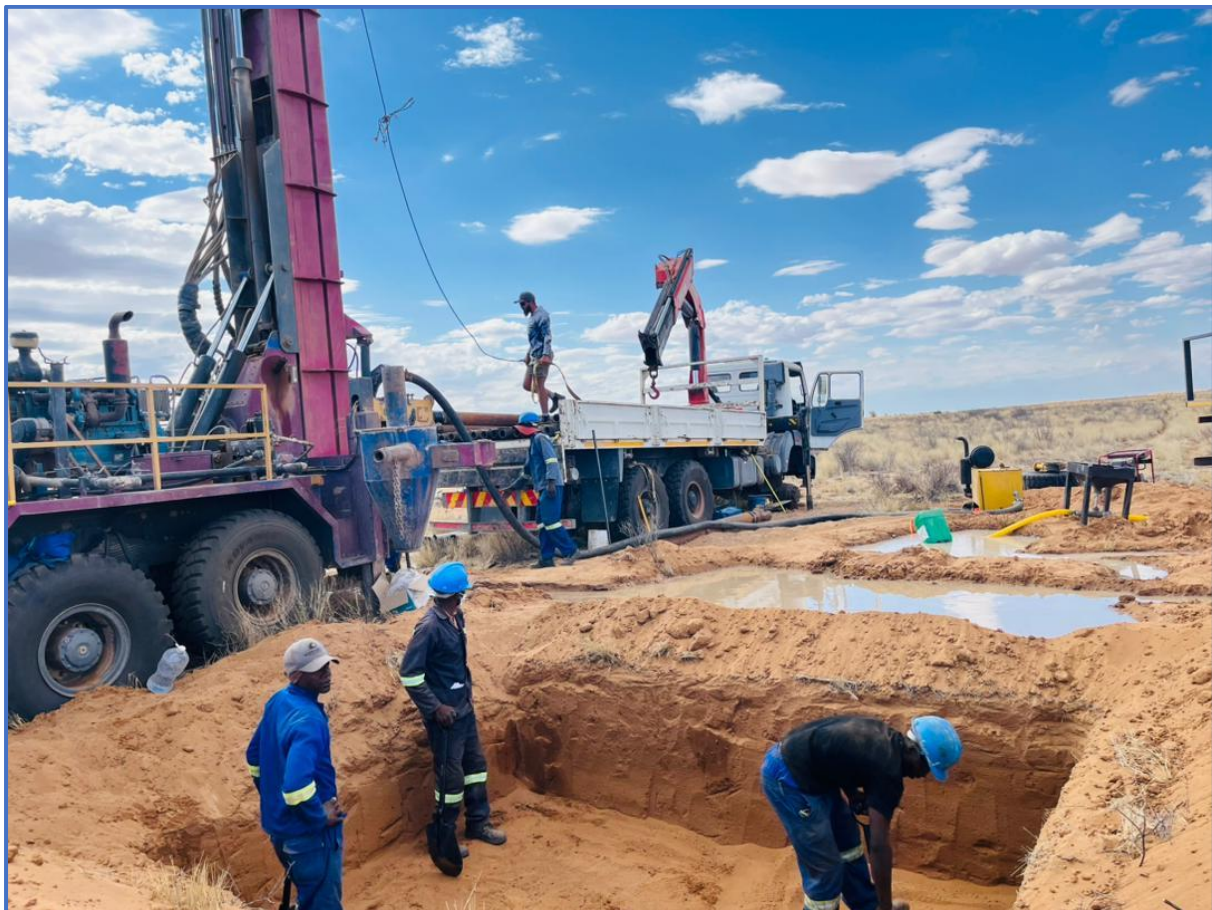
Figure 3: Photo of drilling operations underway
