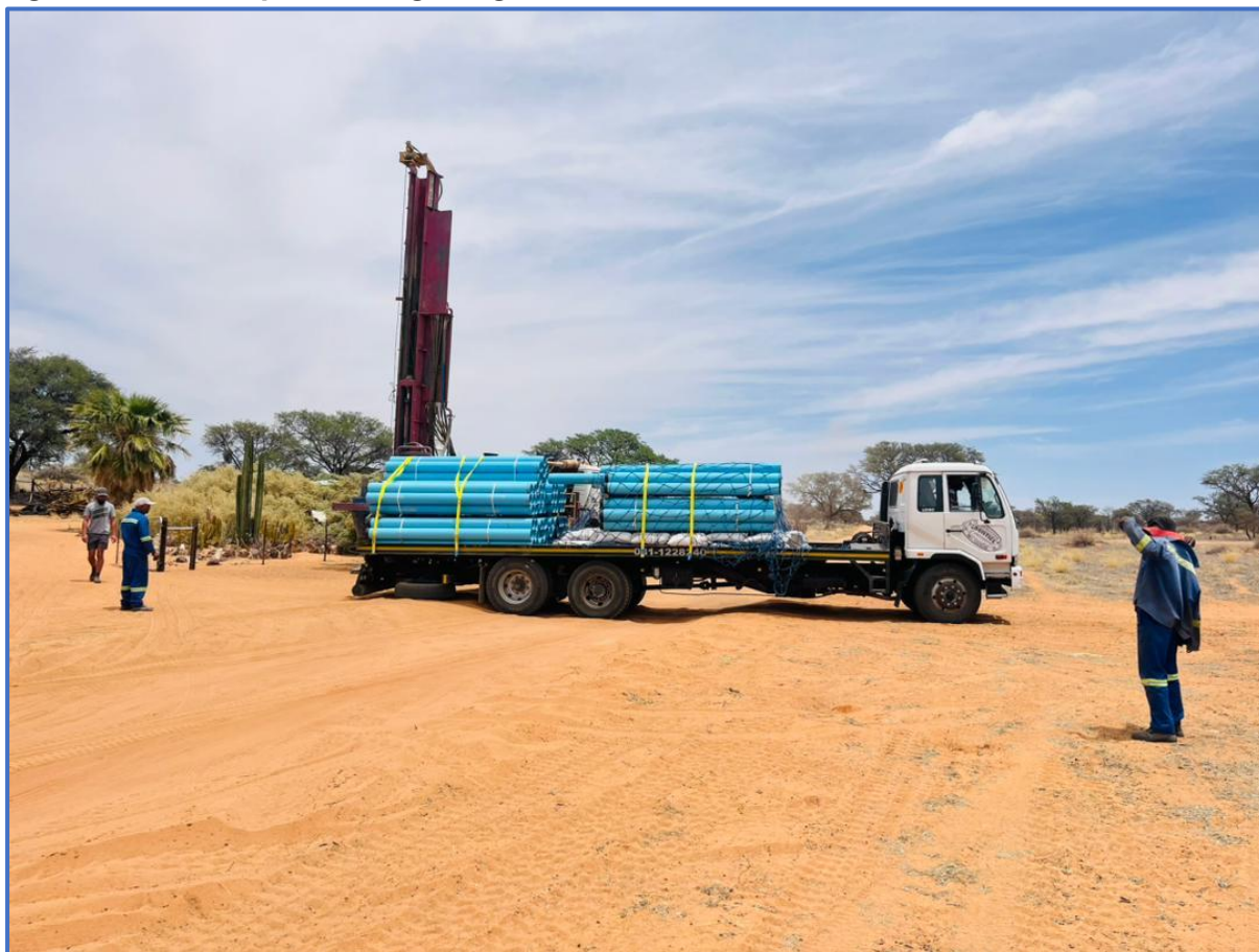
Figure 4: Photo of special casing being delivered
