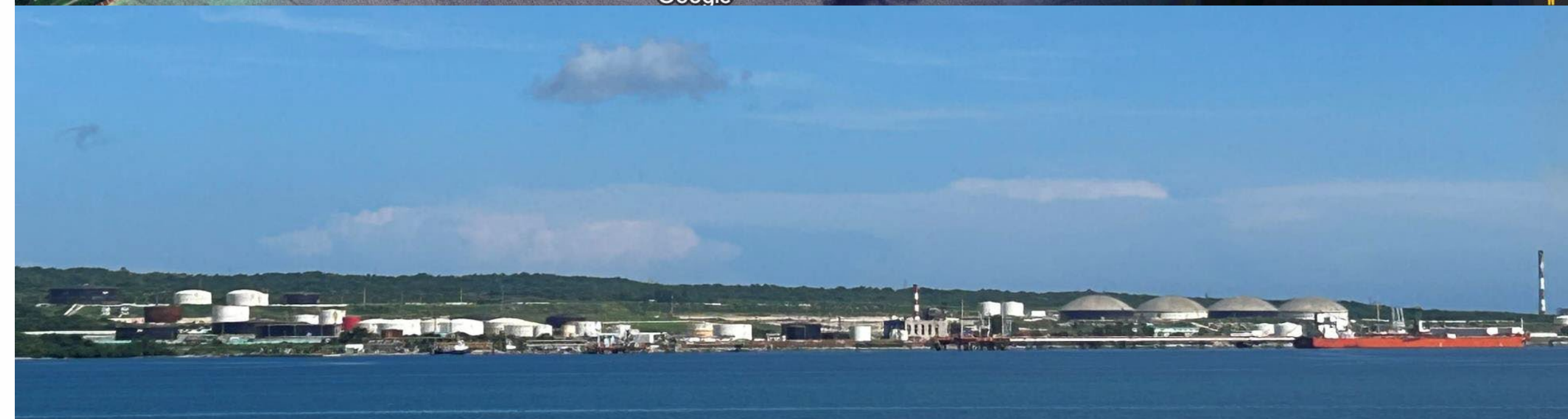
Matanzas Port and Refinery facilities as seen from the bay
