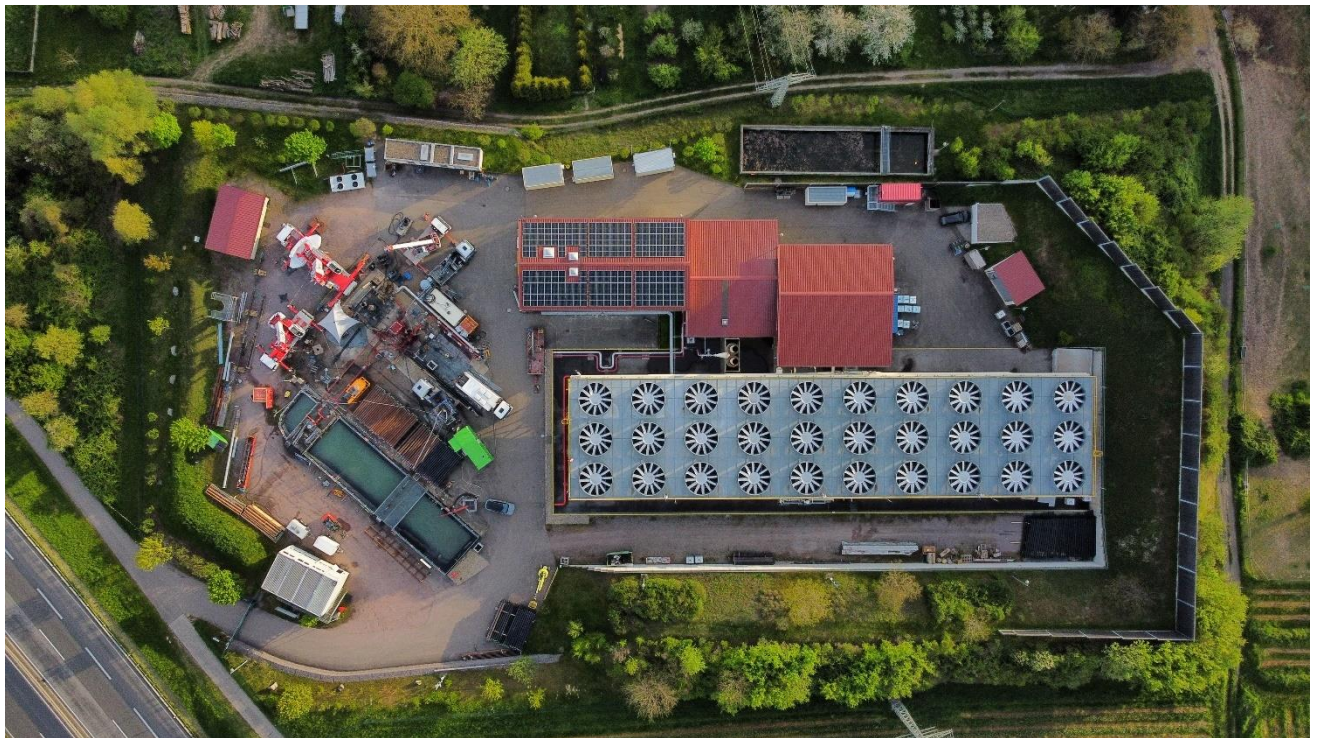
Figure 7 Aerial photograph of Vulcan's Natürlich Insheim Geothermal Plant.
