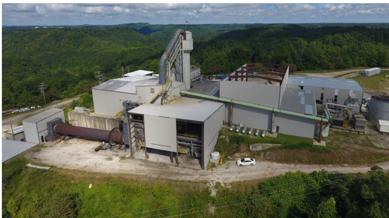
Figure 4 Aerial Overview of the Facility
