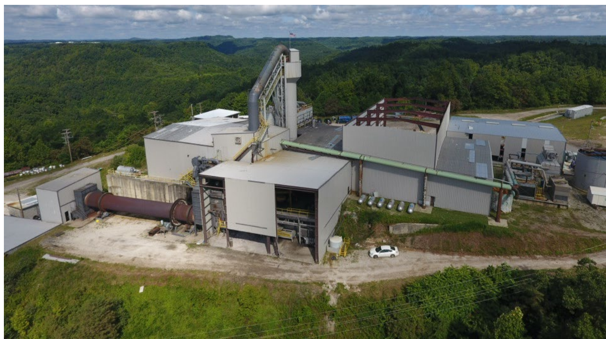
Figure 4 Aerial Overview of the Facility
