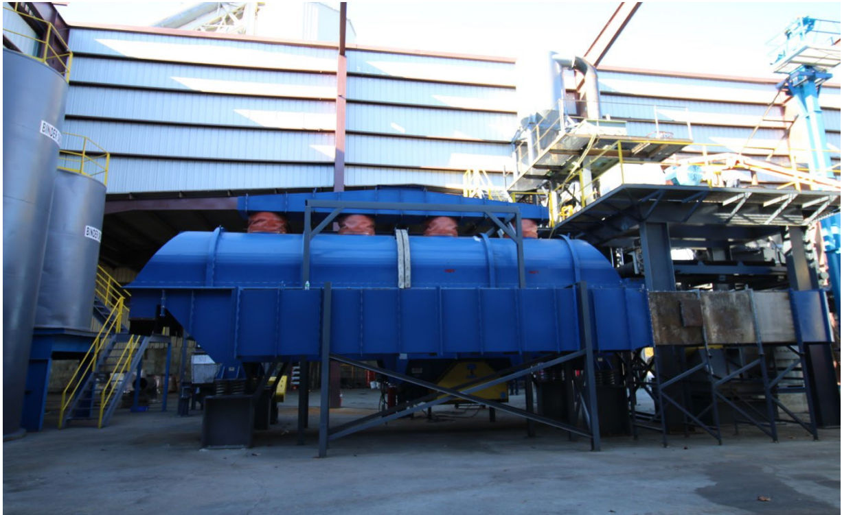
Figure 1: Drying and Baking
