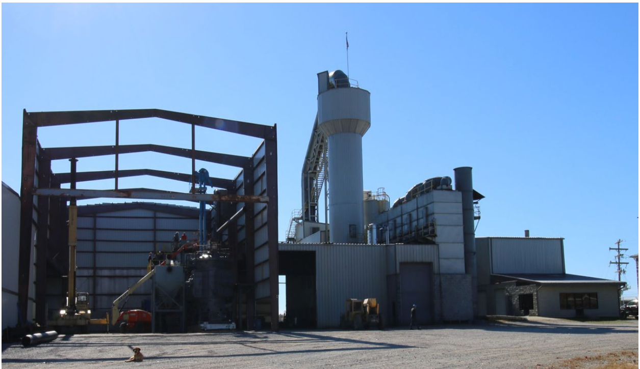
Figure 2: Front view of the Facility
