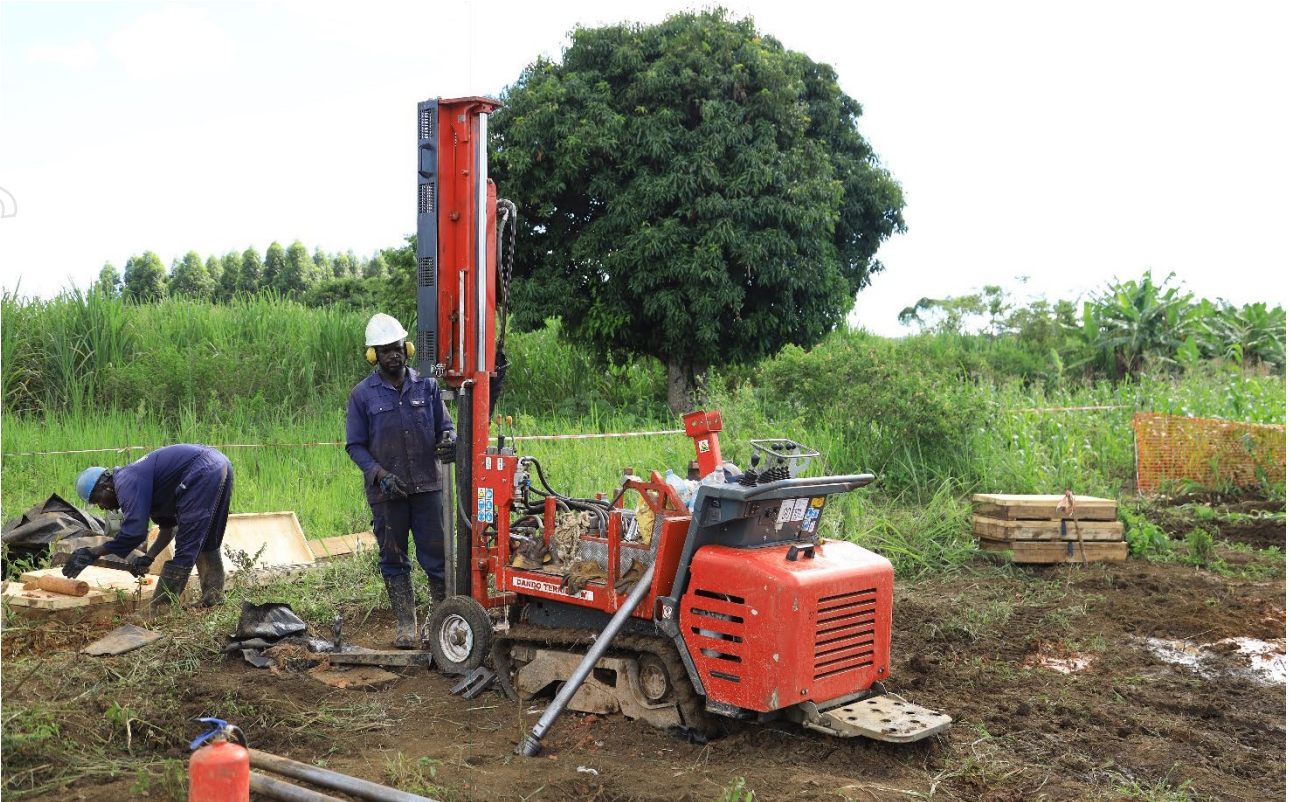
Figure 10: Grade control drilling using a Dando Terrier drill rig.
