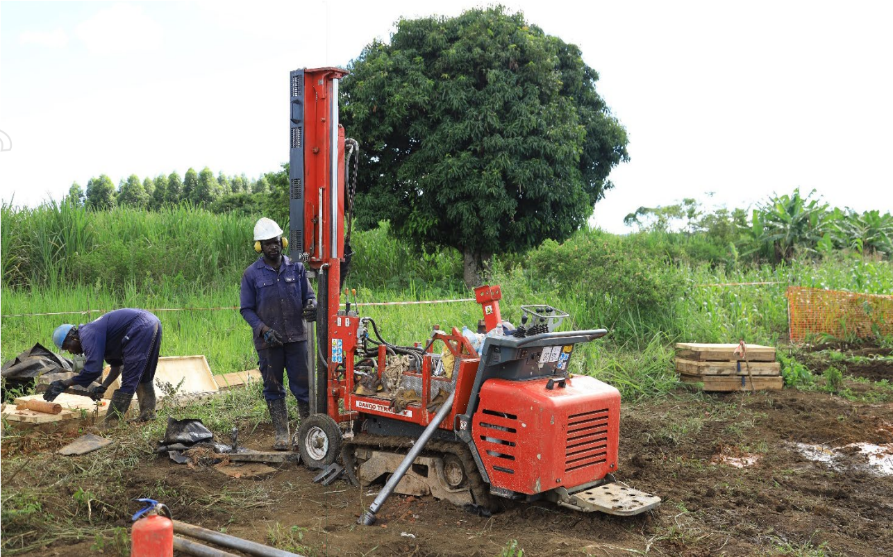
Figure 10: Grade control drilling using a Dando Terrier drill rig.
