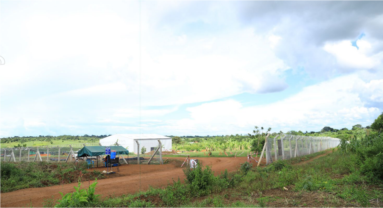
Figure 8: Makuutu Stage 1 Demonstration Plant site secured with perimeter fence.
