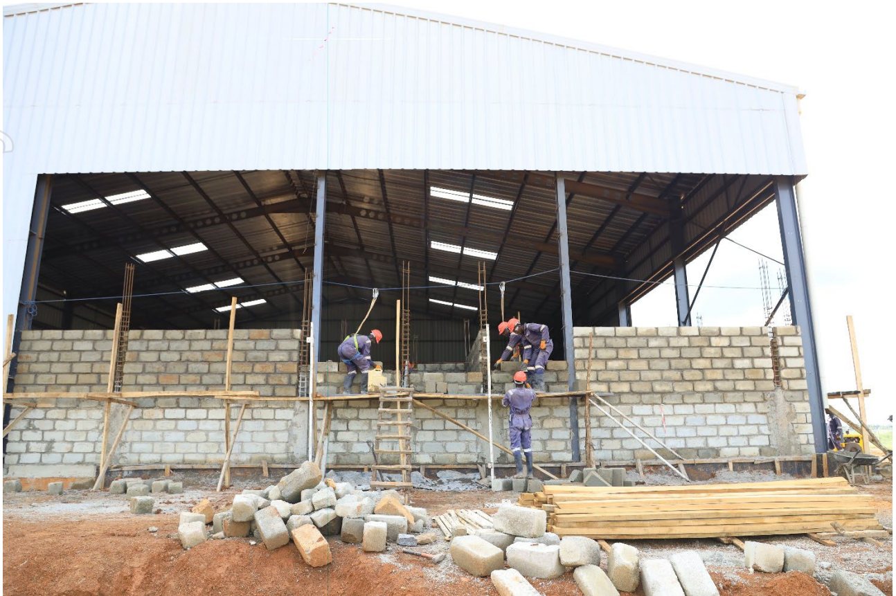
Figure 4: Construction of Technical Facility laboratory brickwork.
