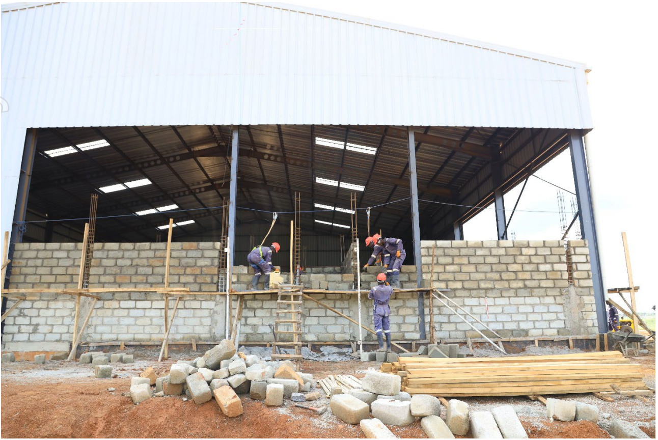
Figure 4: Construction of Technical Facility laboratory brickwork.
