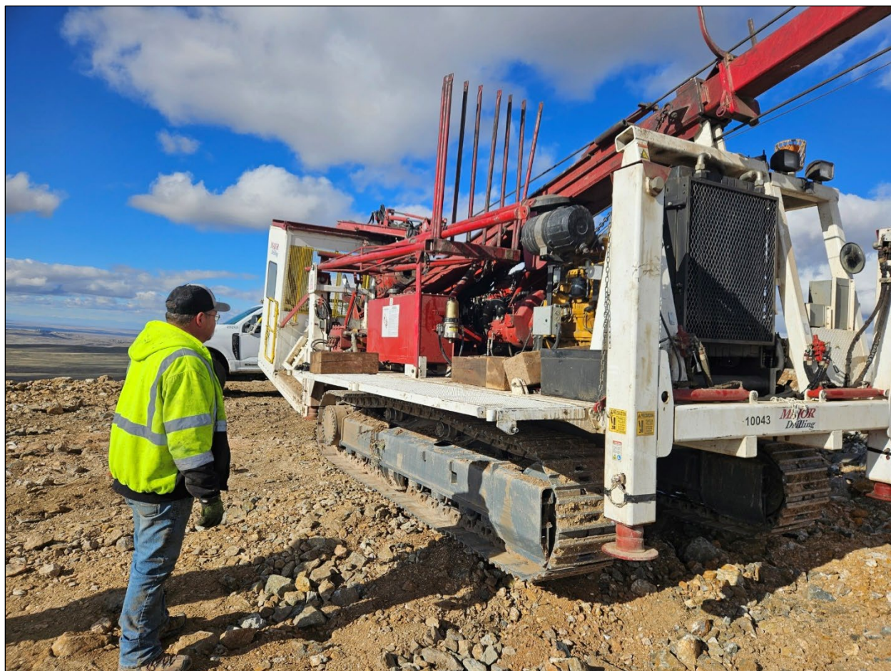
Figure 1: Major Drilling Drill Rig Positioned on a Drill Pad
