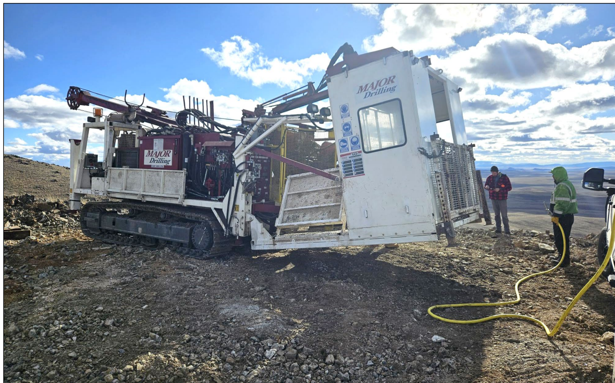
Figure 5: Drill Rig Setup
