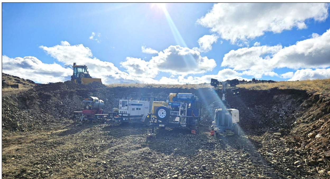
Figure 6: Support Equipment Mobilised to Black Mountain
