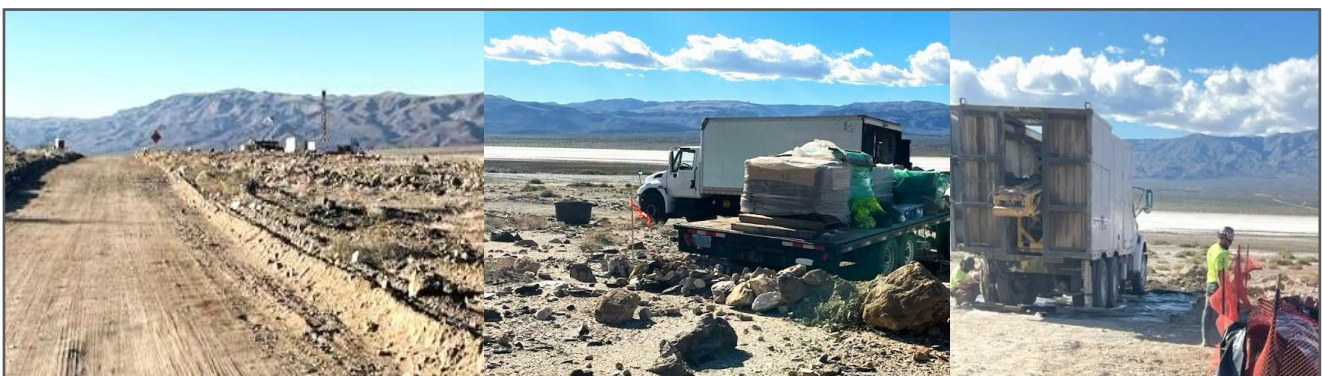
Figure 1: Drill rig – Photos at the first drill hole at the Liberty Lithium Brine Project
