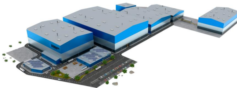
Figure 12: San José Lithium Chemical Processing Facility
