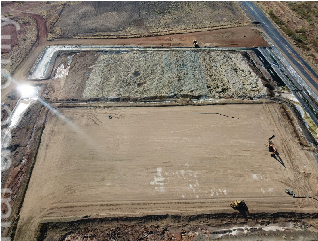
Figure 2. Great Australia Heap Leach Pad 6, stacked and under leach. Pad 5 prepared for receiving material in the foreground.
