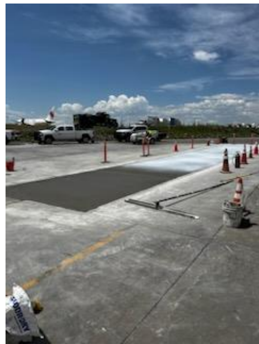
Figure 2. Completed full depth replacement slab
