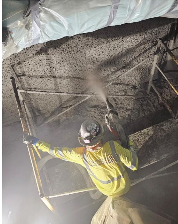
Figure 9. Shotcrete being sprayed onto wall with little dust and rebound.
