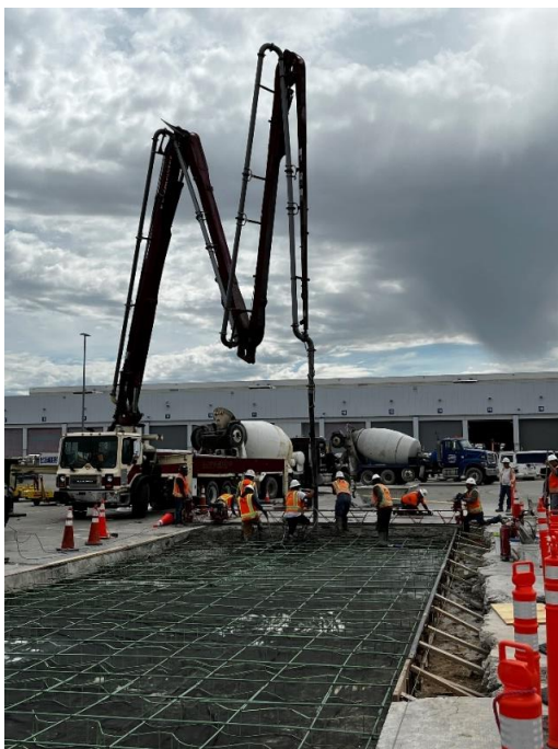
Figure 1. Concrete being replaced in full depth slab
