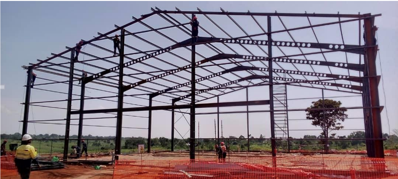
Figure 3: Makuutu Technical Facility frame structure erected.
