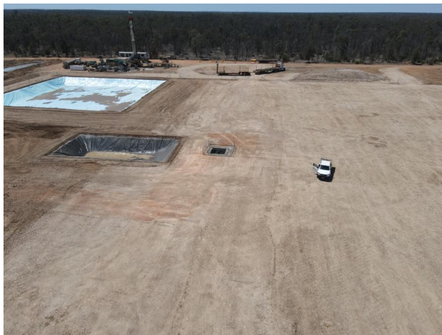
Site work for Daydream-2
