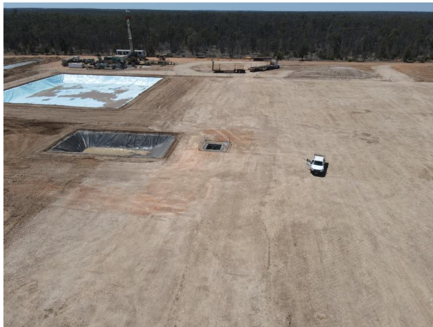
Site work for Daydream-2
