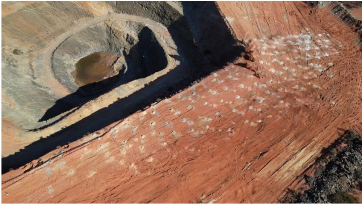
Figure 1: First blast at Selkirk's North wall
