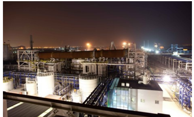
17,000 tpa Jiangsu Lithium Carbonate Plant
