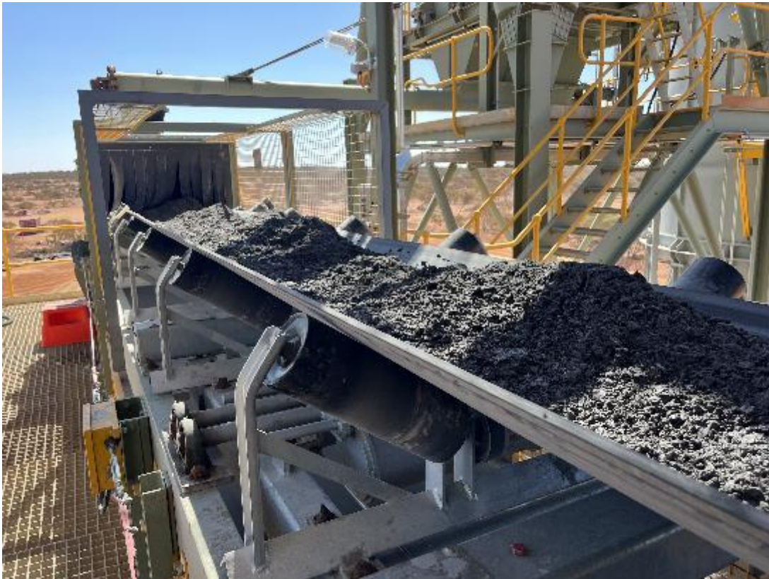
Figure 10 – Picture showing paste cake on the Abra paste-fill plant feed belt to the paste mixture (photo 4 October 2023).
