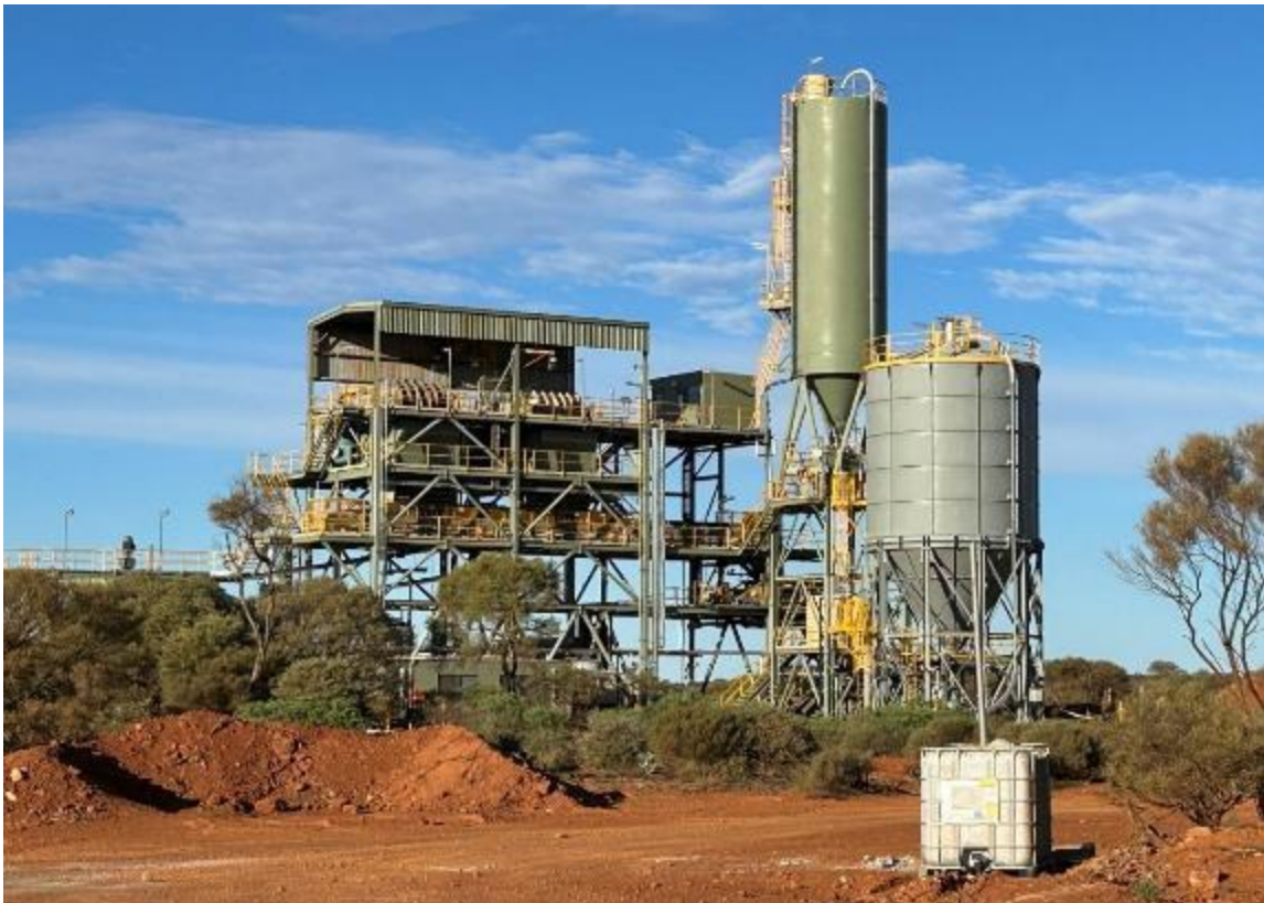
Figure 9 – Abra paste-fill plant.
