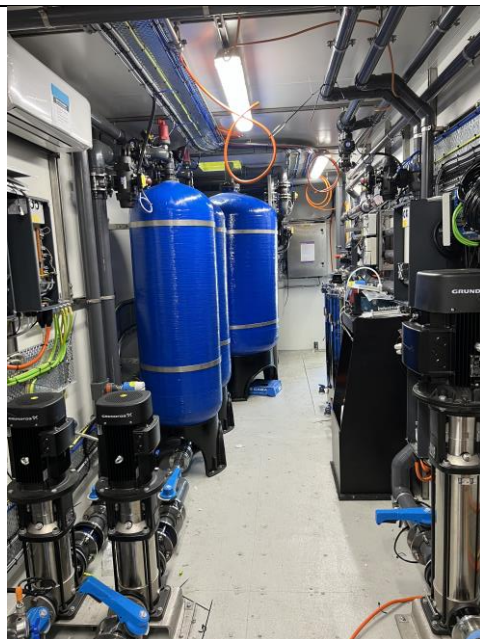
Image 2) De.mem Containerized Membrane Based Water Treatment Plant
