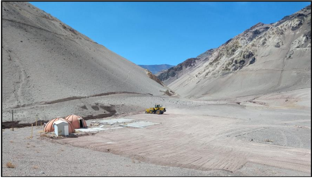
Figure 18: Toro Camp Groundwork Complete
