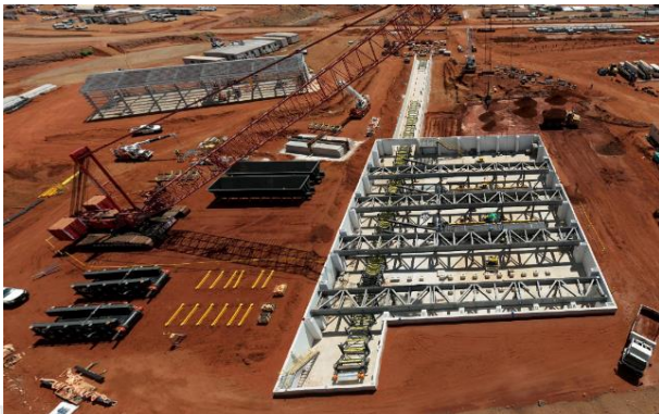
Unloading shed feeder installation
