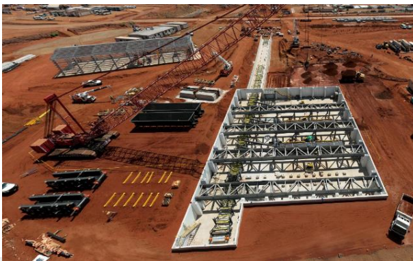
Unloading shed feeder installation
