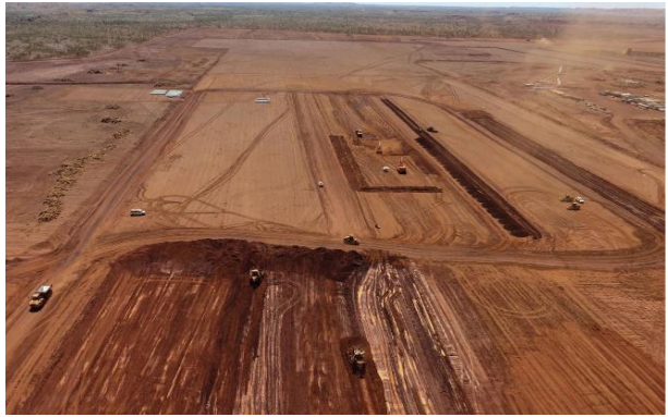
Stockyard earthworks progressing
