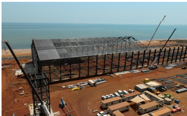
Port ore storage shed steel erection
