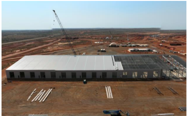
Road train truck maintenance facility
