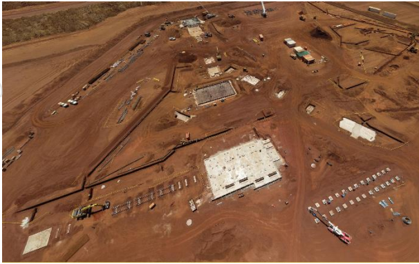
Ken's Bore crushing plant pad concrete works
