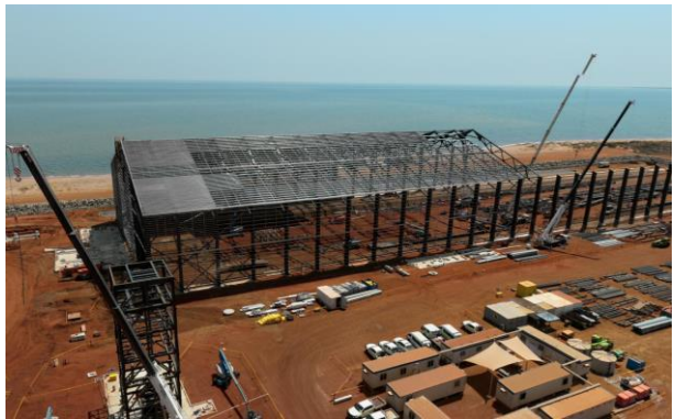
Port ore storage shed steel erection
