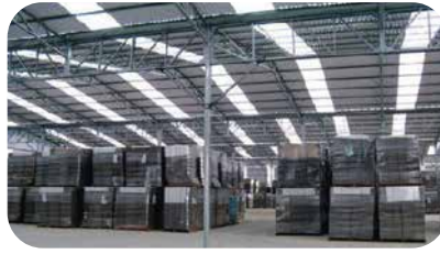
Transparent roof project to reduce lighting usage.
