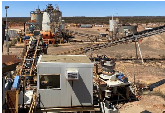
Laverton Processing Plant. May 2023
